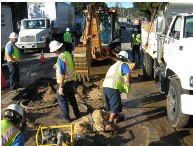
To address physical leakage, service line repairs, leak repairs, and line replacements occur on an ongoing basis. The City has a multi-year service line replacement program to eliminate all polybutylene service lines, which was a widely used material between the early 1970s and the late 1980s until it was found to be defective. To date, 5,442 or over half of all polybutylene service lines on the system have been replaced with copper lines.
