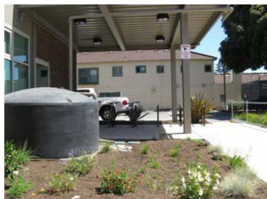
**Demonstration Rain Water Harvesting System and Overflow to Rain Garden at Ecology Action**
