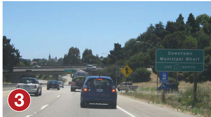
Sign location OK. RECOMMEND requesting Caltrans to change message to "Downtown Santa Cruz / Left Lanes".
