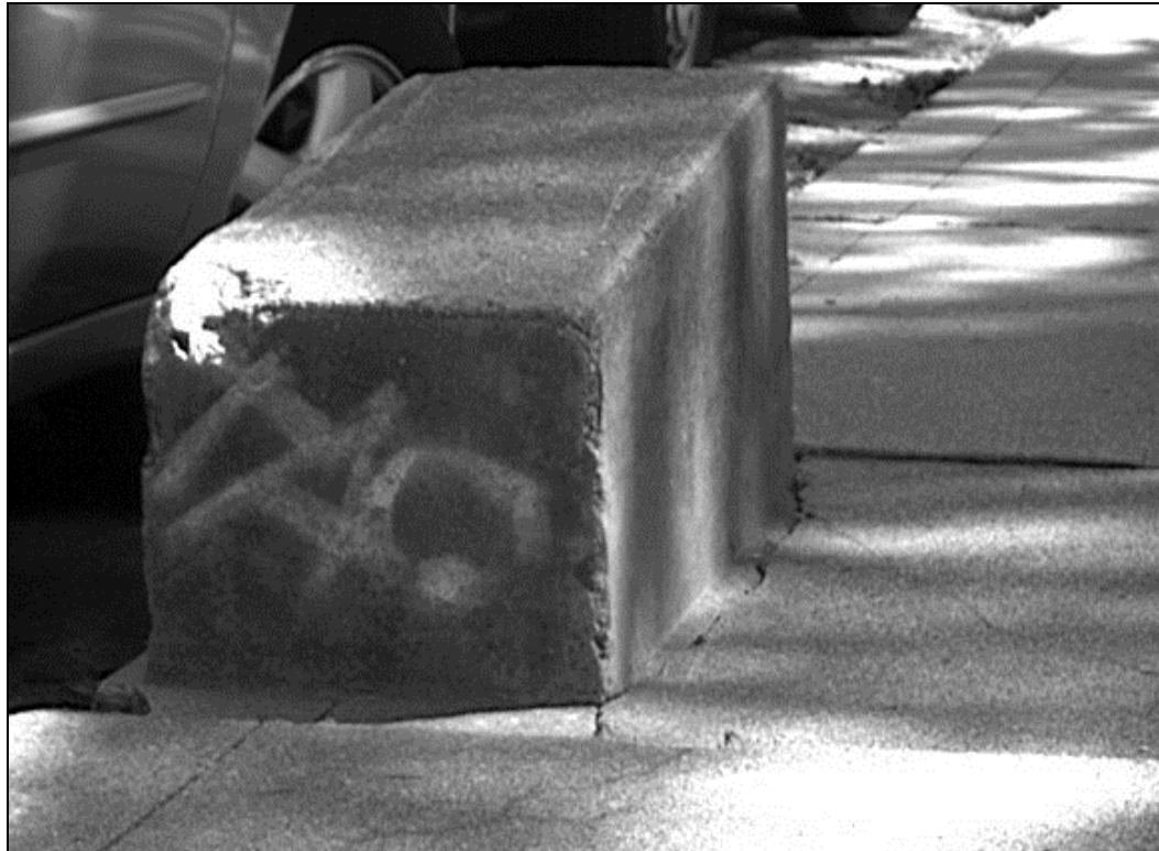
Mounting Block at 123 Green Street.
