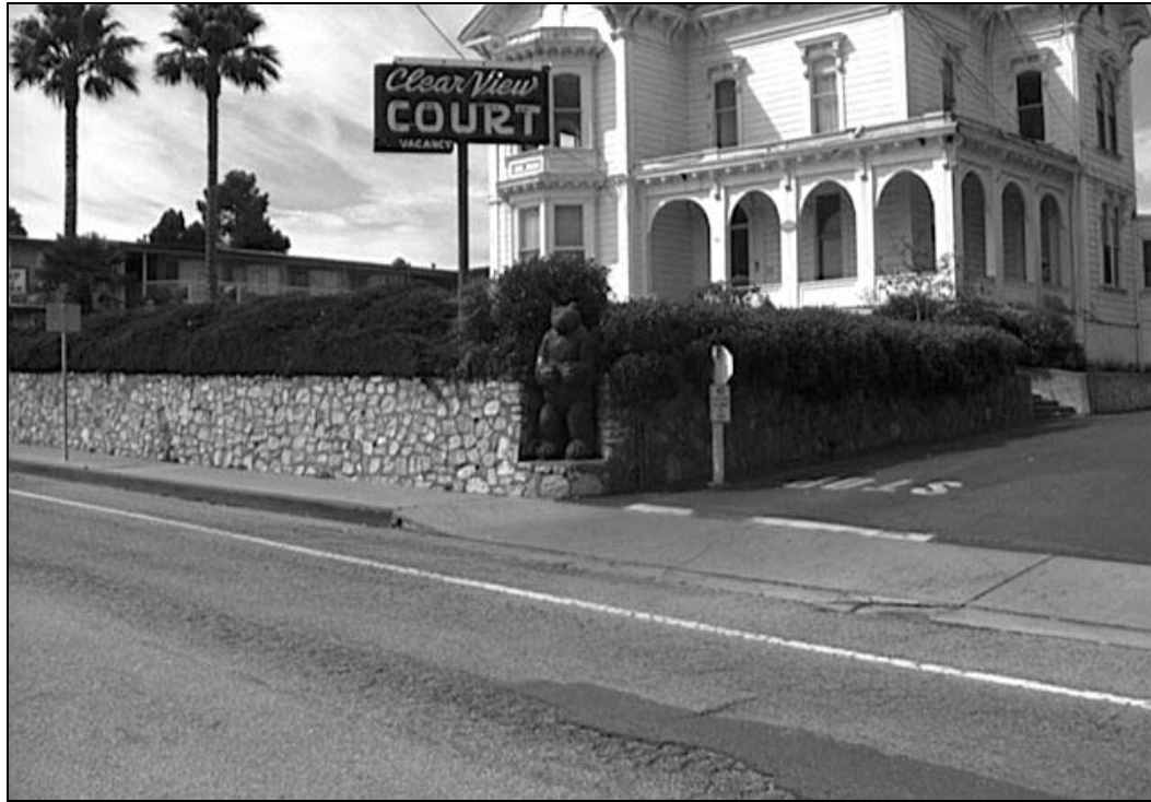
Lynch House Wall located at 174 West Cliff Drive.
