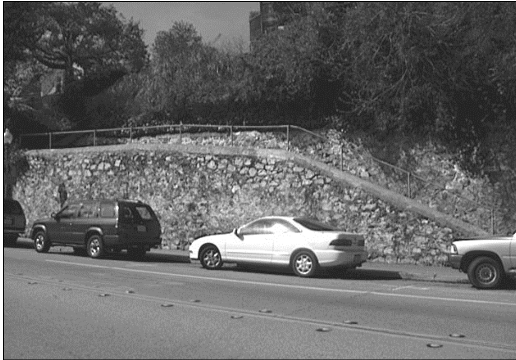
Pratchner Wall and Stairs located on Walnut Avenue.
