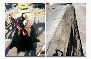
The West Cliff sinkhole has been completely filled in. Phase 2 work continues including work on the piers and is expected to conclude by the end of next week with final paving. Phase 3 work which will place more rock in the cove around the outside of the sinkhole area for greater stabilization is still a ways off as we must go through a preliminary design process within the regulatory/jurisdictional framework.
