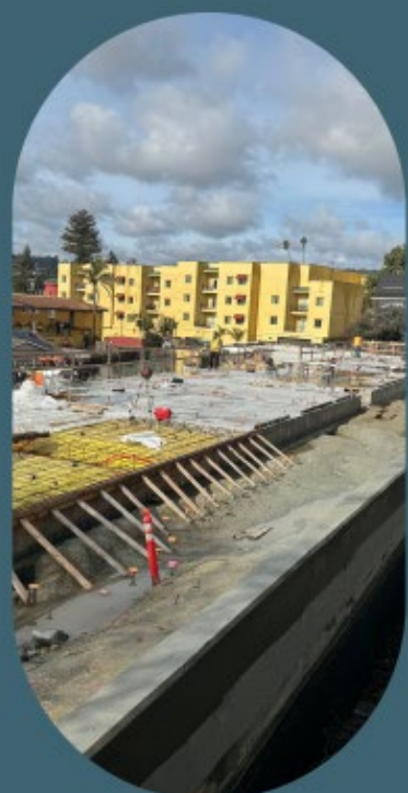
100% affordable Jessie St Apartment Construction 2024
