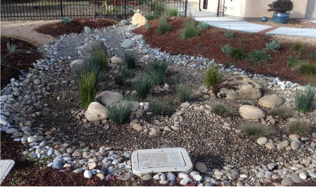
Green stormwater infrastructure (source: City of Santa Cruz)
