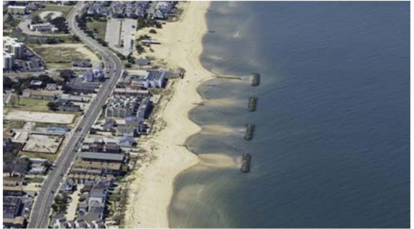
Example of constructed breakwaters
