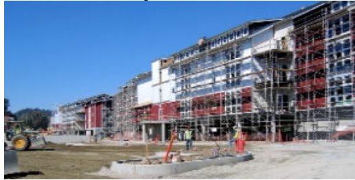
Tannery Lofts During Construction
