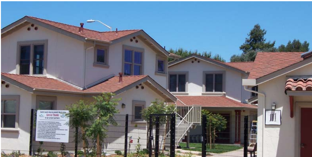
Nueva Sol Supportive Housing
