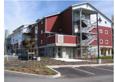
Tannery Lofts Completed
