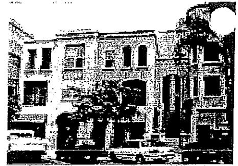
Multiple family residential: over ground floor commercial. Architecture incorporates building modules, offsets, bays, porches and balconies to minimize scale.
