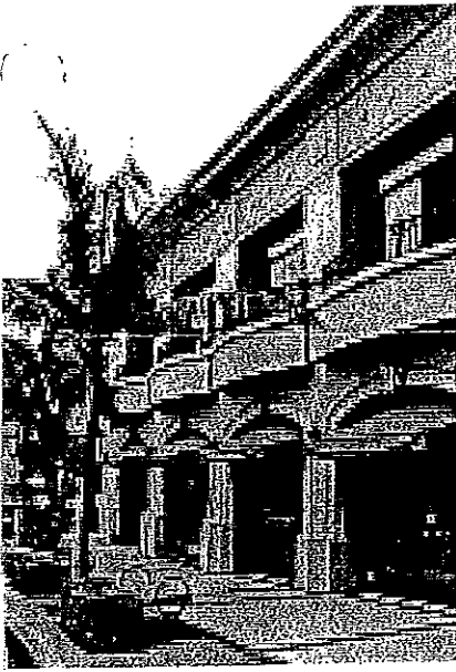
New Commercial development utilizes traditional architectural elements including cornices, balconies, arches and metal railings, and wall decoration. Pedestrian amenities include awnings, benches, landscaping, and textured paving
