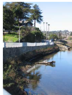
Contract 3 – Laurel Street Extension
