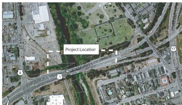
Highway One Bridge Project
