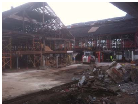
Historic Tannery Building during Phase Two Renovation
