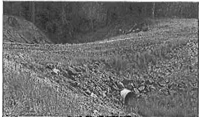
Culvert Work DFG photo by JoAnn Dunn
