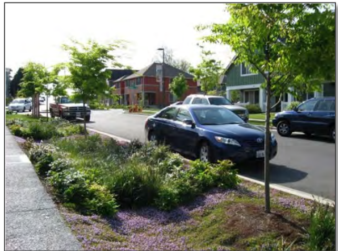
Pervious concrete sidewalk and bioretention swale (Source: US EPA [Wikimedia Commons])
