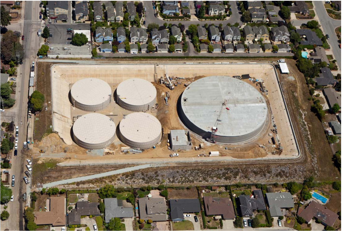
Bay Street Reservoir
