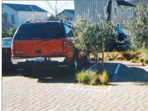
High-quality, permeable brick paving.
