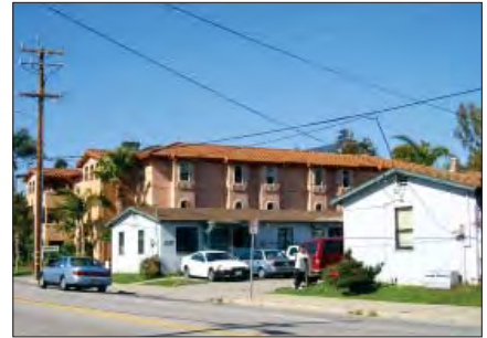
This motel and one-story apartment building are near Broadway.
