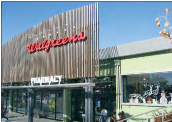
Externally illuminated signs integrated with a building's architectural details.
