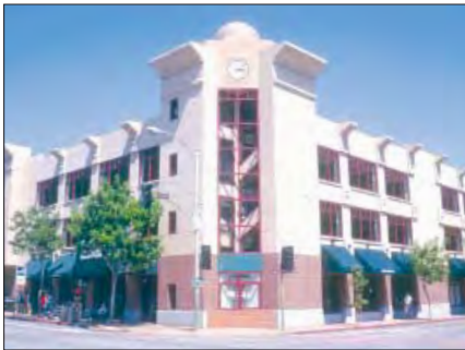
Parking structures lined with retail stores will enhance the character of Ocean Street.
