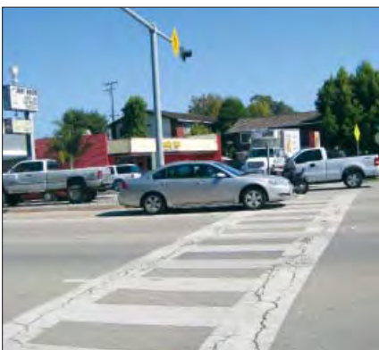
An unprotected crosswalk at Leonard Street has an overhead flashing light to alert drivers that pedestrians may be present.
