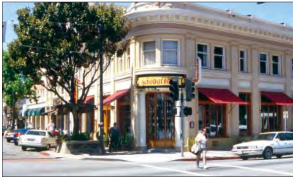
Columns and a recessed bay accent an entrance.
