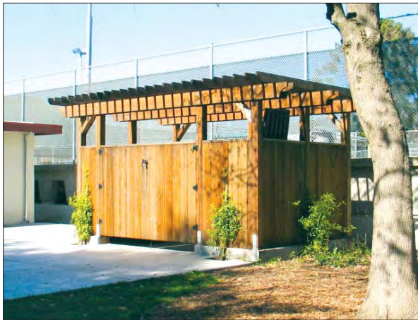
Screened trash enclosure.
