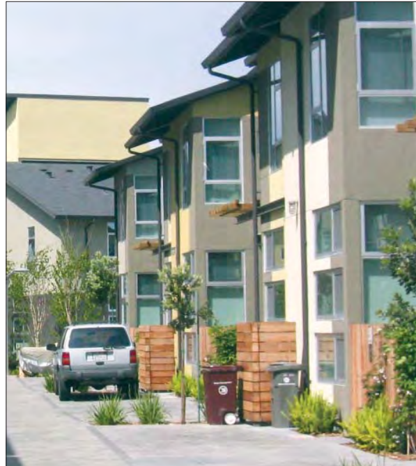
Trash enclosures can complement the architecture of a building.
