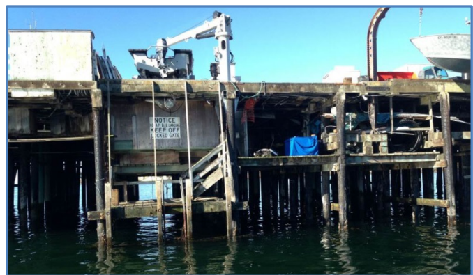
The Wharf Operations dock utilizes a 3-ton crane to launch Wharf and SCFD Marine Rescue equipment.
