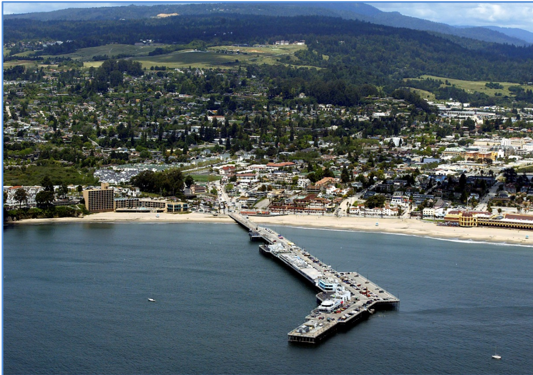
Constructed on a base of over 4,400 Douglas-fir piles, the Santa Cruz Wharf is the longest timber-supported structure in the United States. The Wharf Master Plan proposes a 2.5 acre expansion for public access, recreation, and engagement with the Monterey Bay National Marine Sanctuary.
