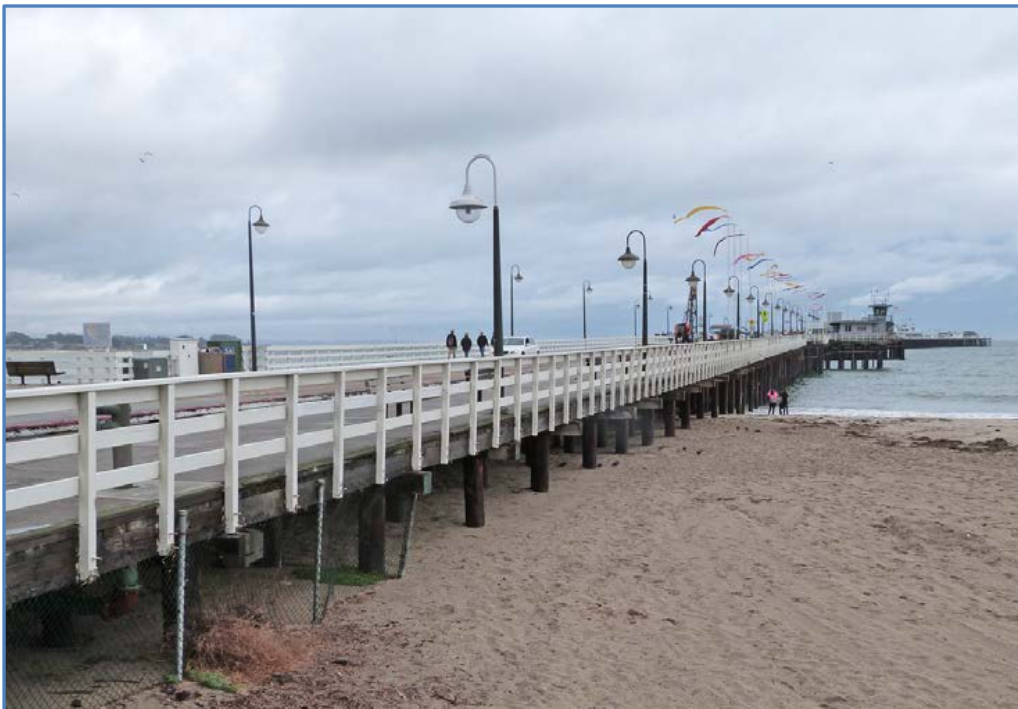
The 1914 Wharf was approximately 4 acres in size. Between the 1950's and 1980's, it was increased by 3.3 acres for commercial uses and parking.
