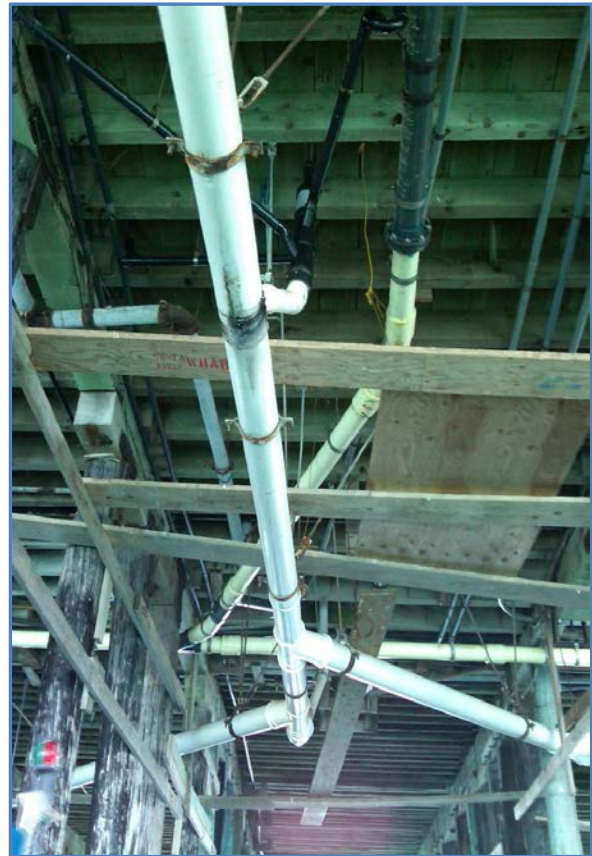
Sewer mains and laterals are in serviceable condition.
