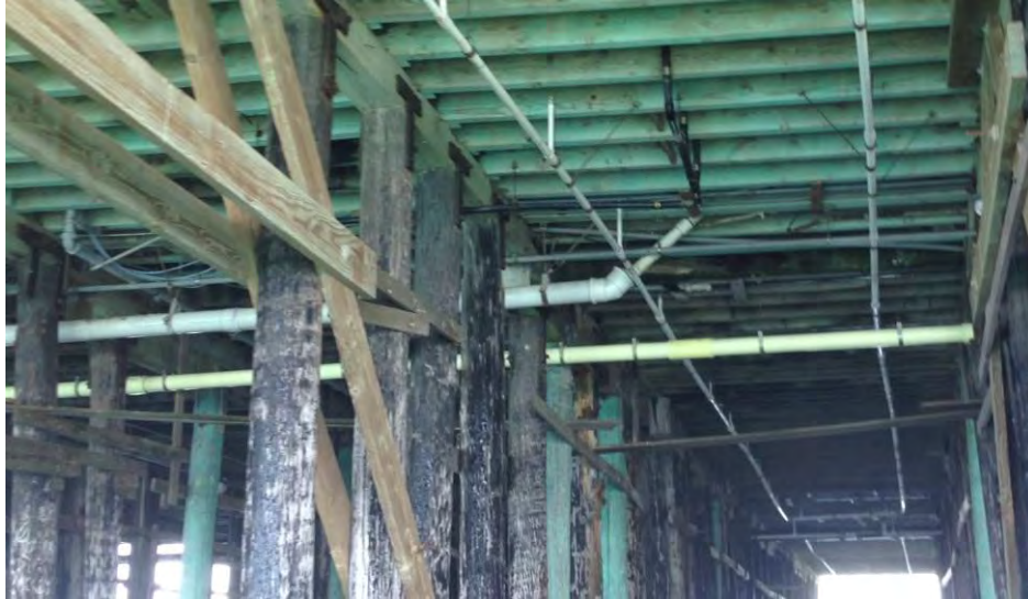
Photo 5-3: Cleanout at High End of Gravity Line
