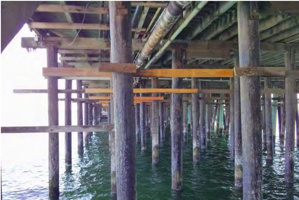
Photo 1-1: Typical Wharf Pile Bent and Structure
