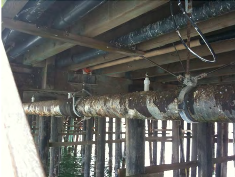
Photo 6-1: 10 Inch Ductile Iron Water Main Near Bent 70
