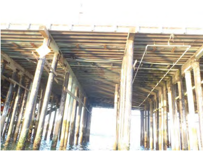
Photo 2-4: Typical Trestle with Parking Bent
