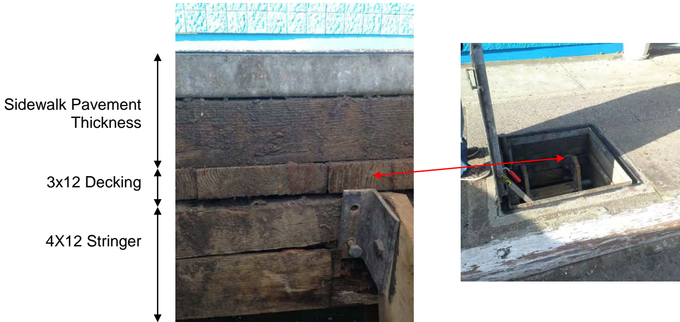
Photo 4-4: Existing Walkway Section at Access Portal
