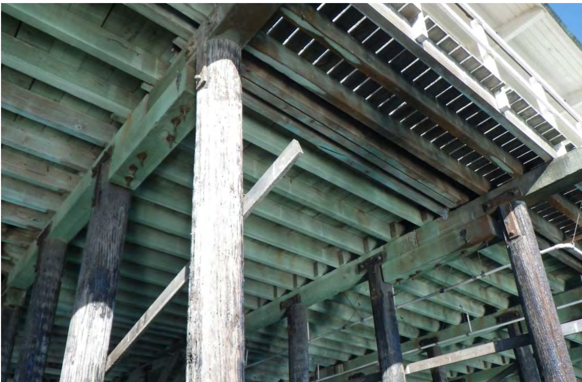
Photo 2-1: Typical Wharf Framing
