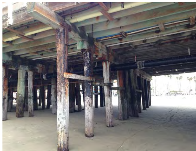
Photo 2-3: Typical Trestle Bent
