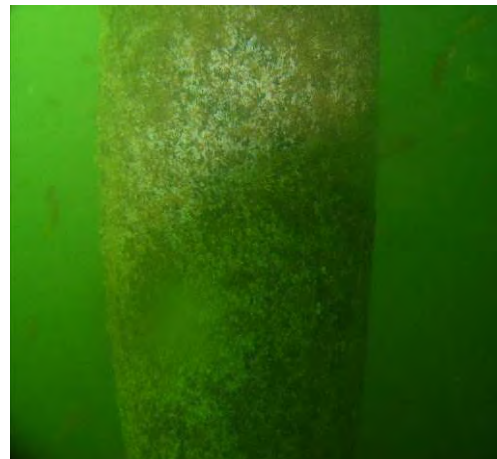
Photo 1-3: Typical non-damaged pile in “excellent” condition
