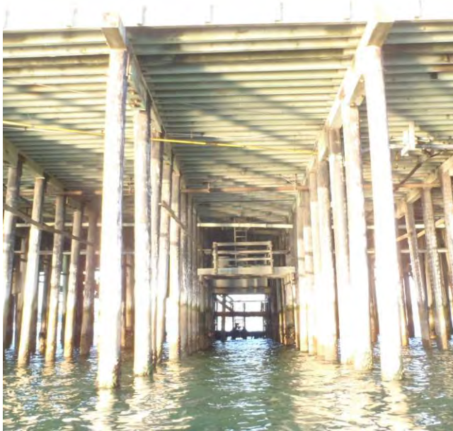
Photo 6-3: Fire Access Portal Platform at Bent 80
