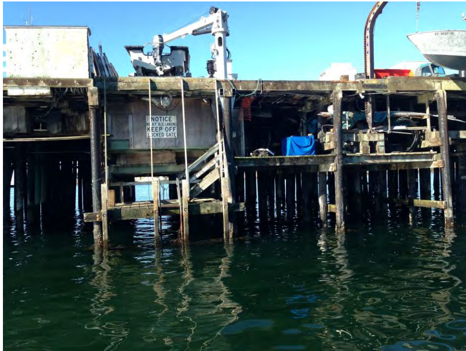
Photo 8-4: Wharf Staff Landing
