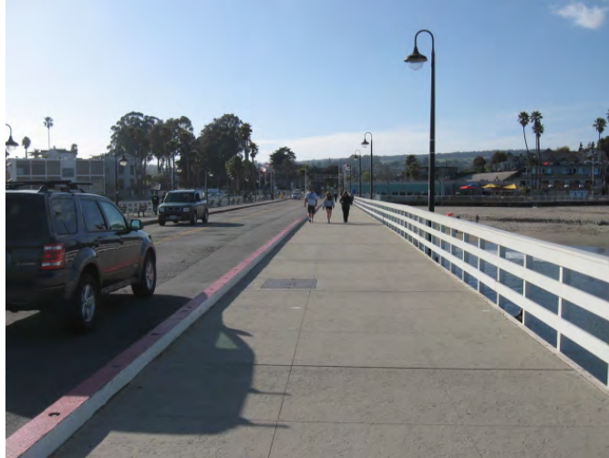
Photo 4-2: Walkway on East Side of Trestle- 13 ft. Width, Stamped Concrete
