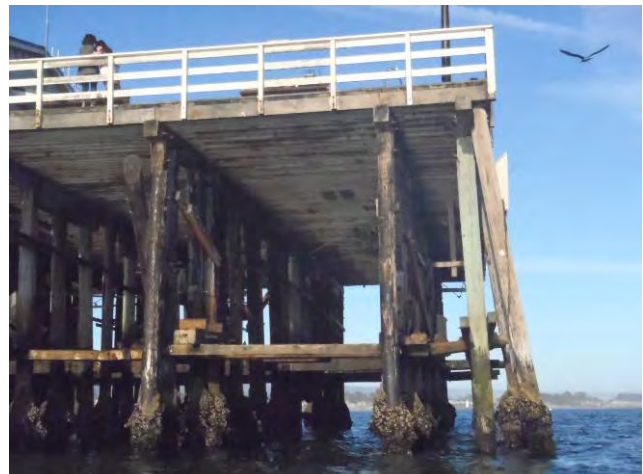
Photo 2-9: Typical End Bent
