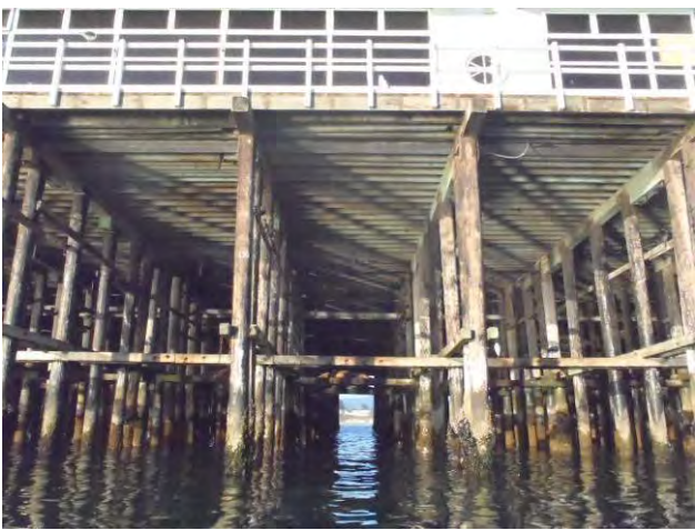
Photo 2-6: Typical East Parking Bent
