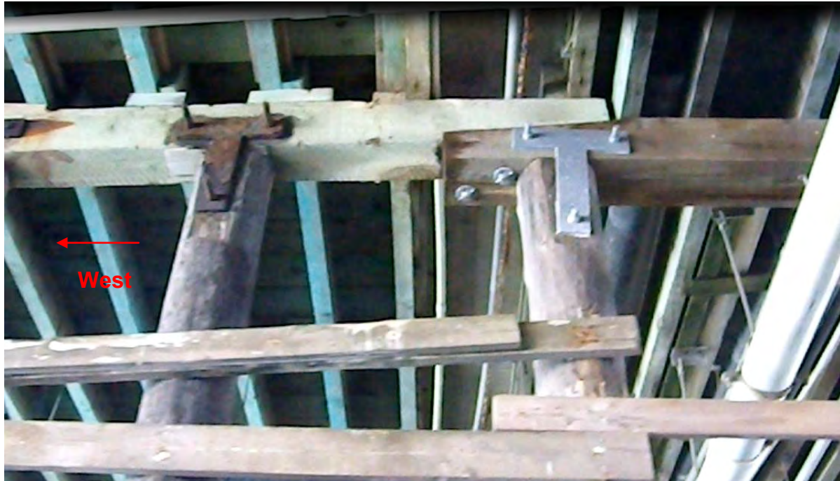
Photo 2-11: Cap/Deck Transition – Bent 99 (Piles 8 and 9)
