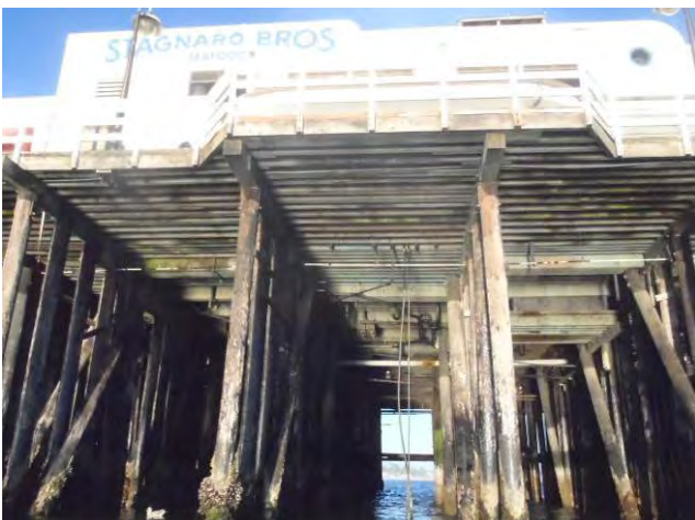
Photo 2-8: Typical Stagnaro's Bent
