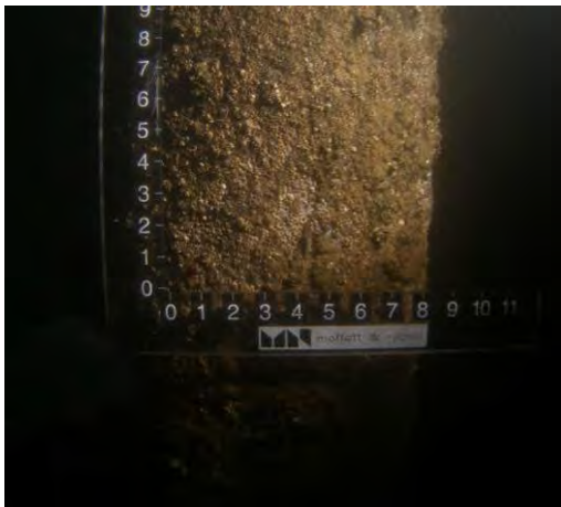
Photo 1-2: Typical non-damaged pile in “excellent” condition
