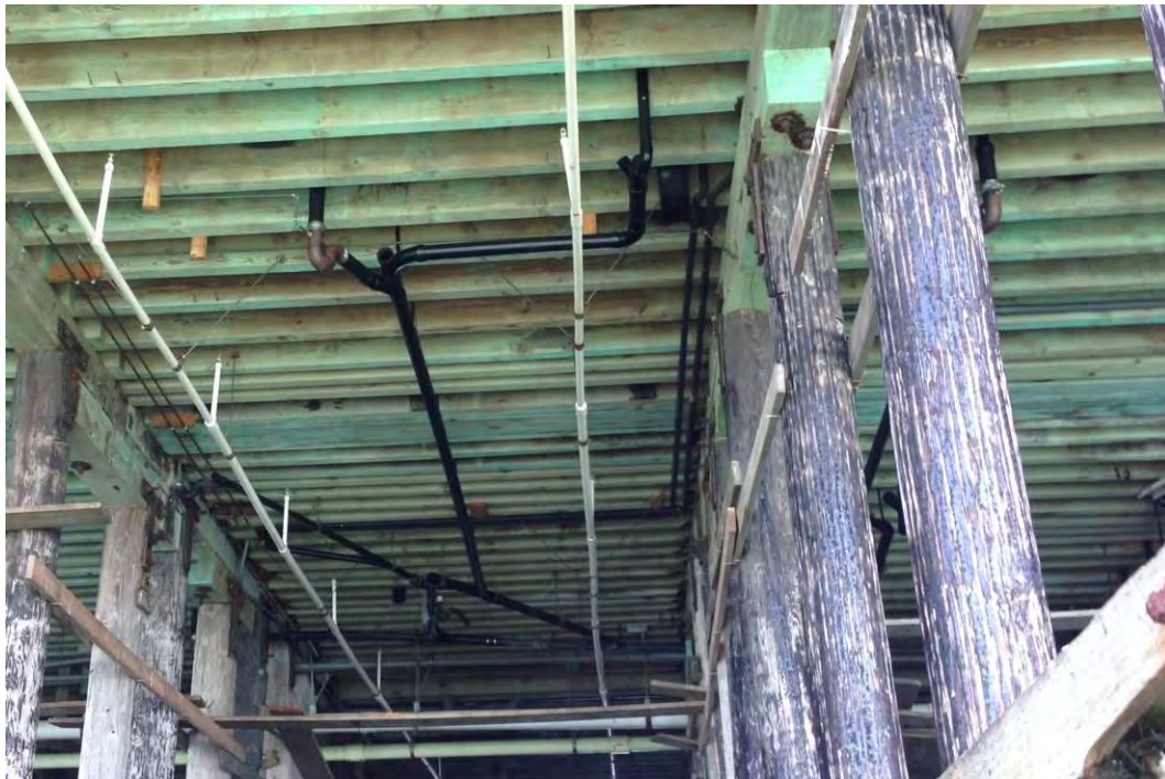
Photo 5-2: Lateral line at Bent 128, New Construction
