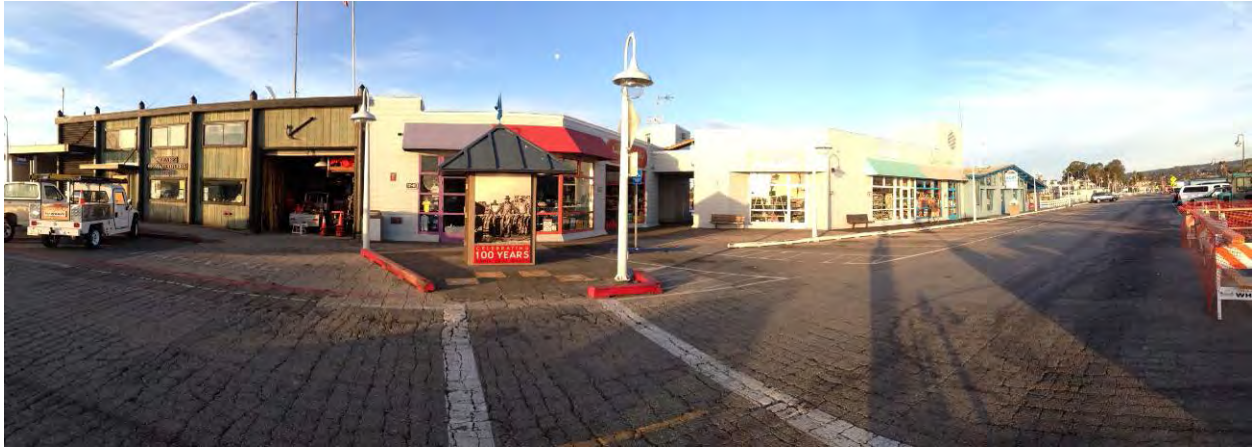
Photo 2-2: Typical topside view of the Wharf
