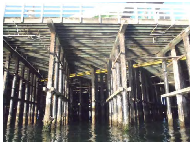
Photo 2-7: Typical Angle Bent
