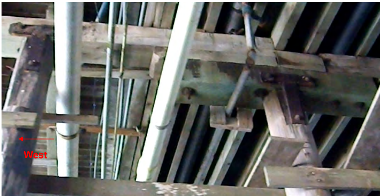
Photo 2-12: Cap/Deck Transition – Bent 125 (Piles 7 and 8)
