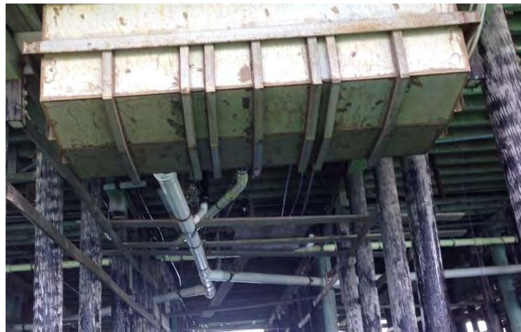
Photo 5-5: Sewer Pump Station at Bent 86
