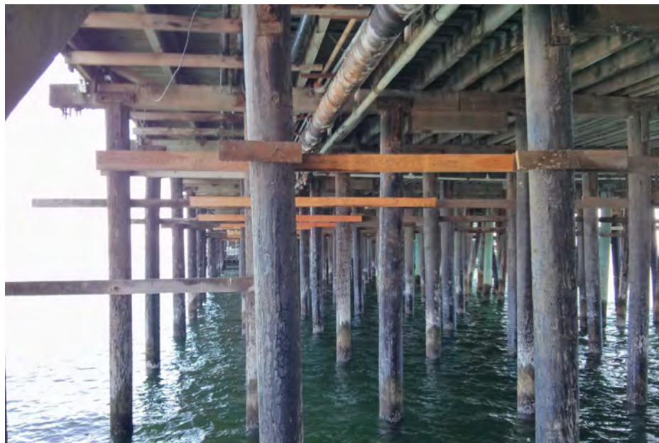
The Wharf is one of the longest pile-supported timber structures in the world and due to the on-going maintenance by Wharf staff continues to be in serviceable and sound condition.
