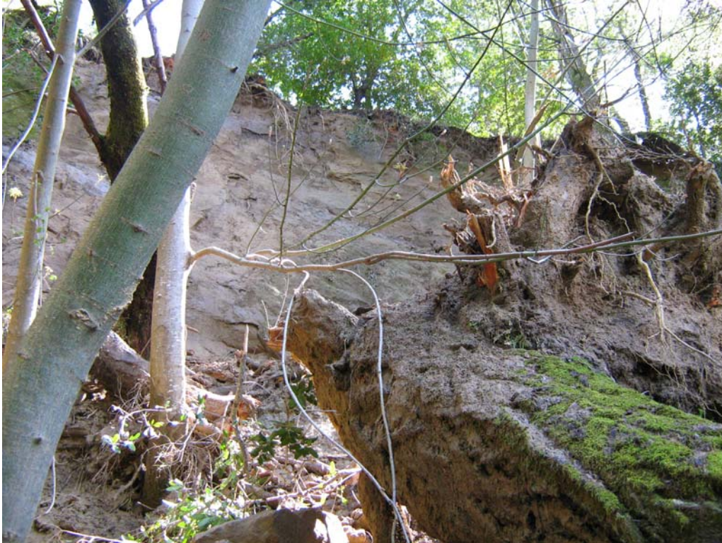
Landslide along Newell Creek Pipeline
