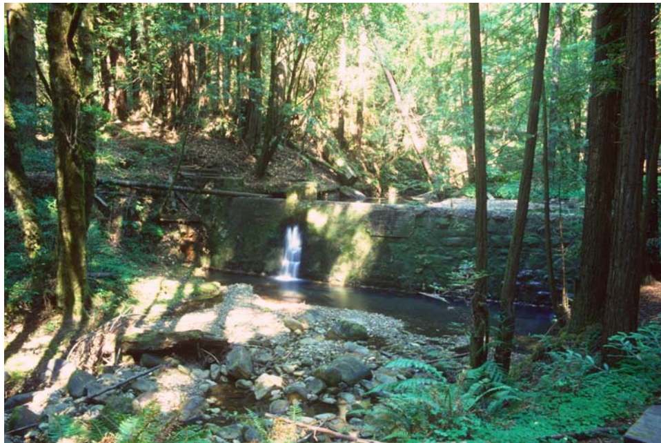
Creek Diversion Structure
