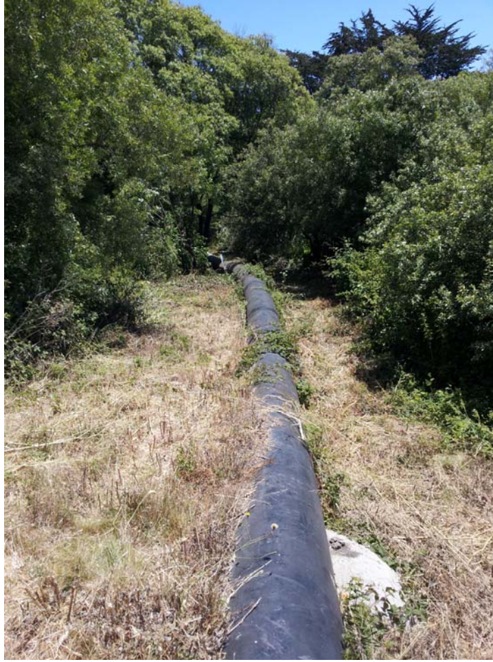
Section Of Phase 3 North Coast Pipeline Project
