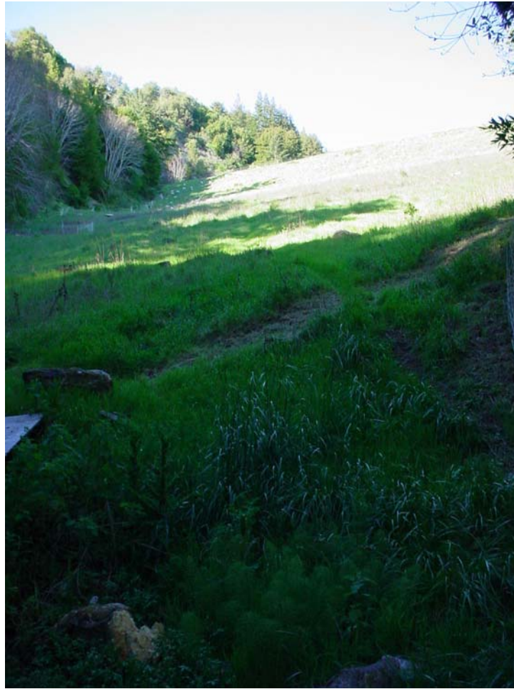
Downstream Face of Newell Creek Dam (view from toe)
