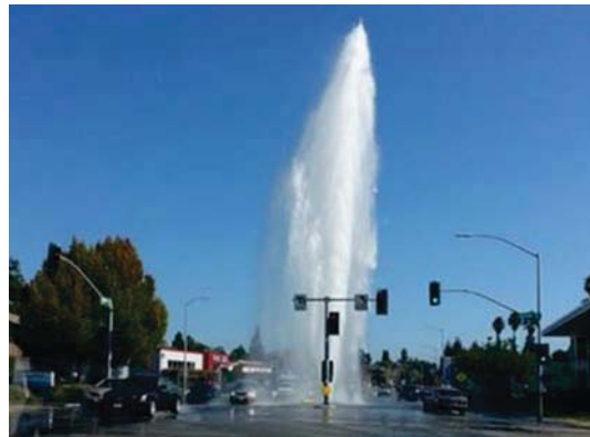
A sheared fire hydrant is a one example of a real water loss
