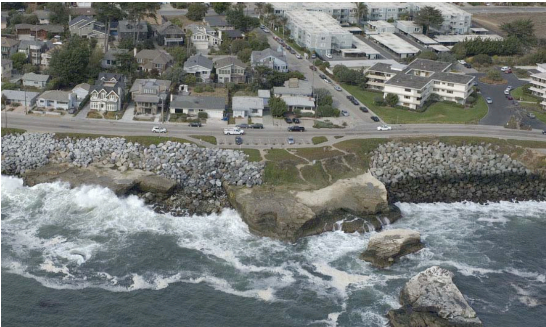
Figure 9. Rip rap along West Cliff Drive (Photo California Coastal Records Project © Kenneth and Gabrielle Adelman)
