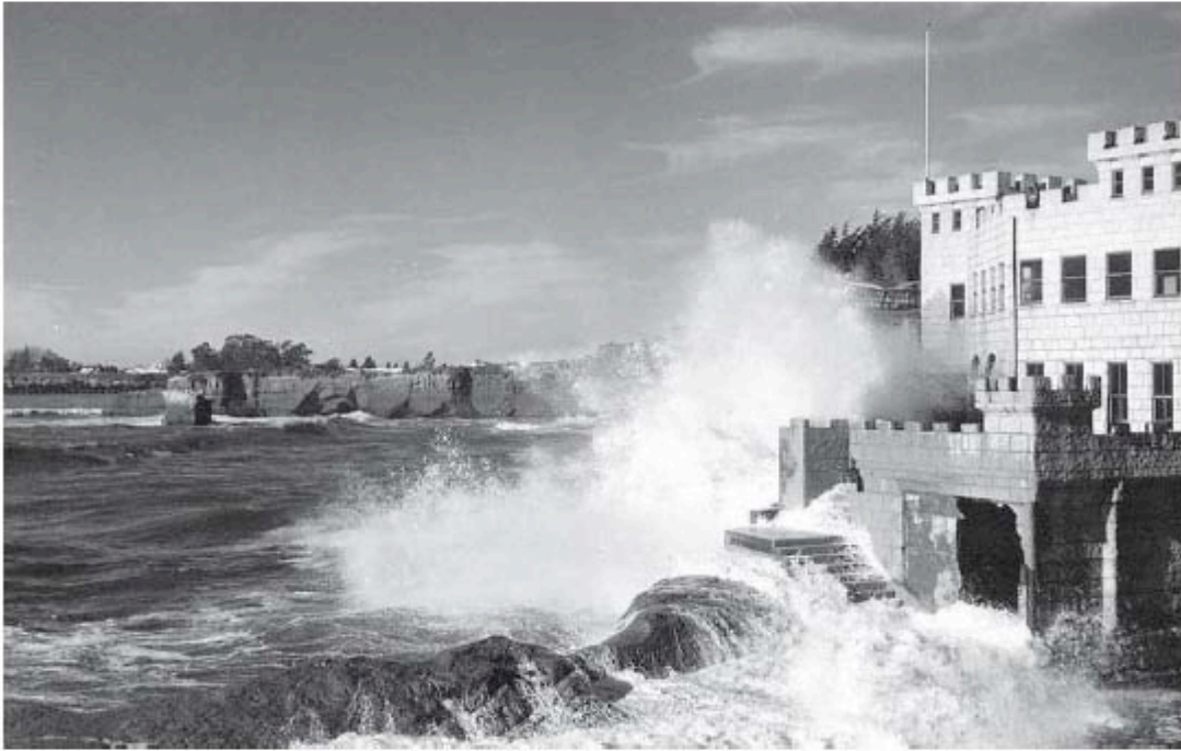
Figure 17a. Castle Beach showing waves attacking bluffs in 1953, before harbor construction. Courtesy of Special Collections, University Library, UCSC.
