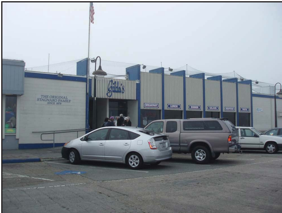
View to the West: Commercial Buildings, built along Wharf roadway.
