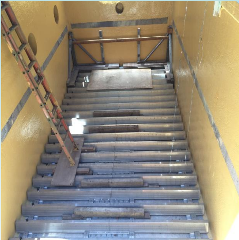
Install stainless underdrains
