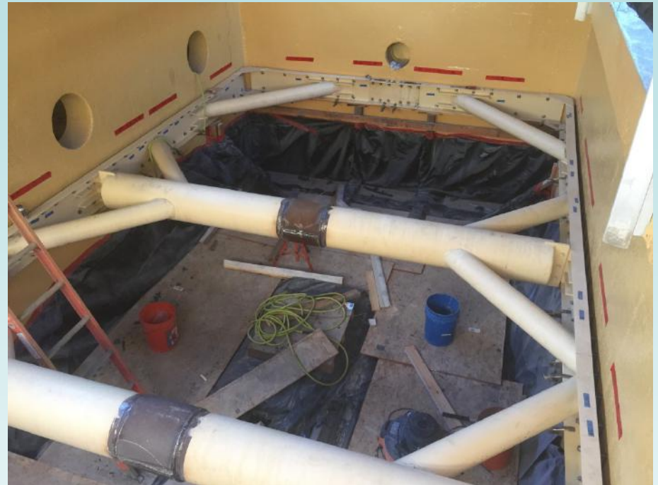
Install structural seismic reinforcement
