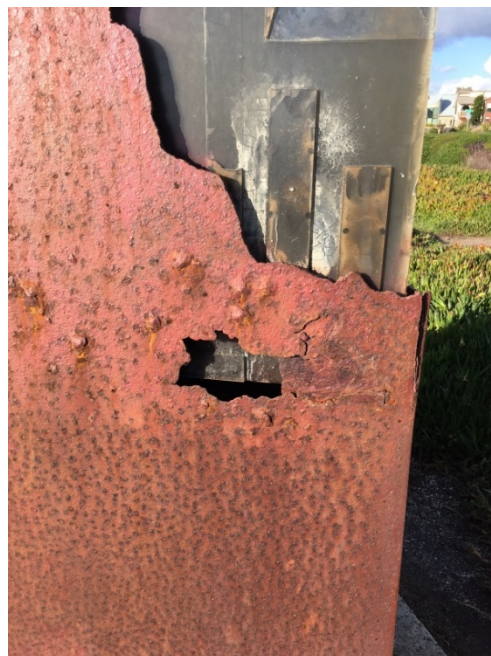
Effects of the marine air and spray have pitted and rusted the piece.
