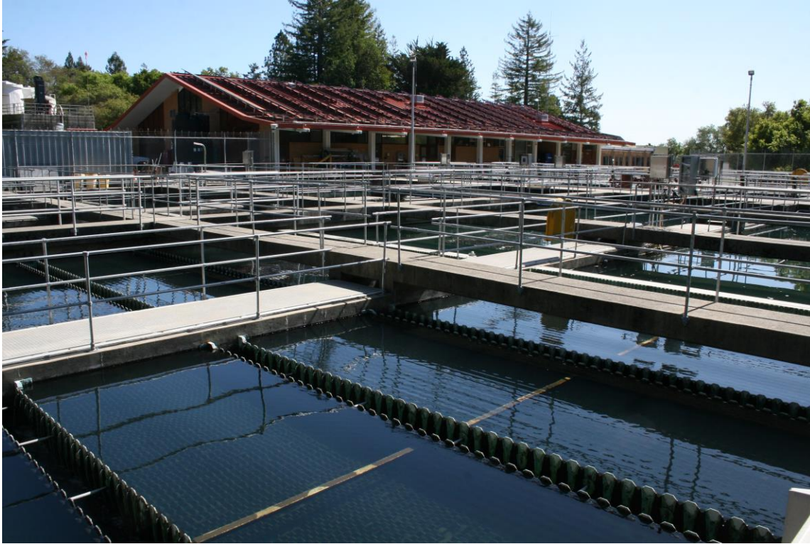
Figure 2: Existing Sedimentation Basins at the GHWTP
