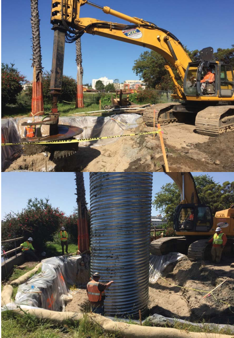
The Branciforte Bike/Pedestrian Bridge and Path under construction. This project will complete the “missing link” to the City’s 5.2 mile San Lorenzo River Levee.
