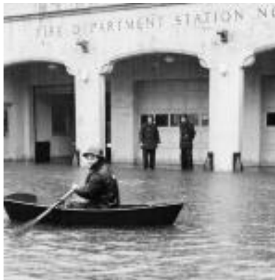
Downtown Fire Station 1955 Flood
