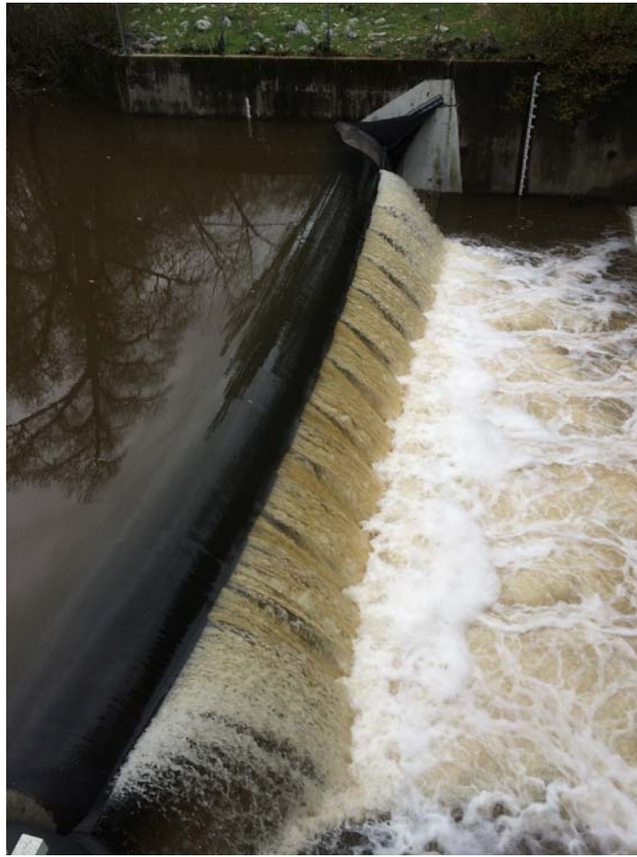
Felton Diversion, Inflatable Dam
