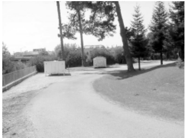
Figure 26 Branciforte Creek Confluence Area - Existing Conditions
