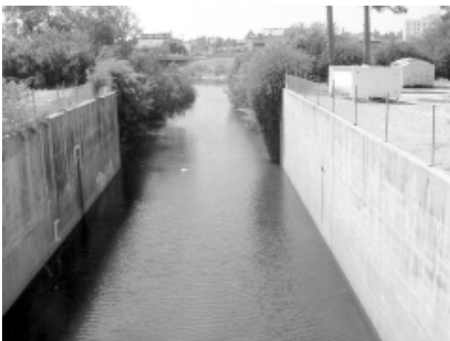
Figure 3 Branciforte Creek Flood Control Channel
