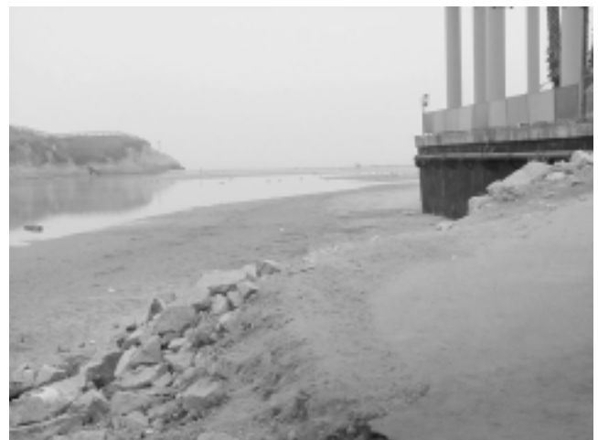
Figure 18 Trestle Bridge Focus Site
