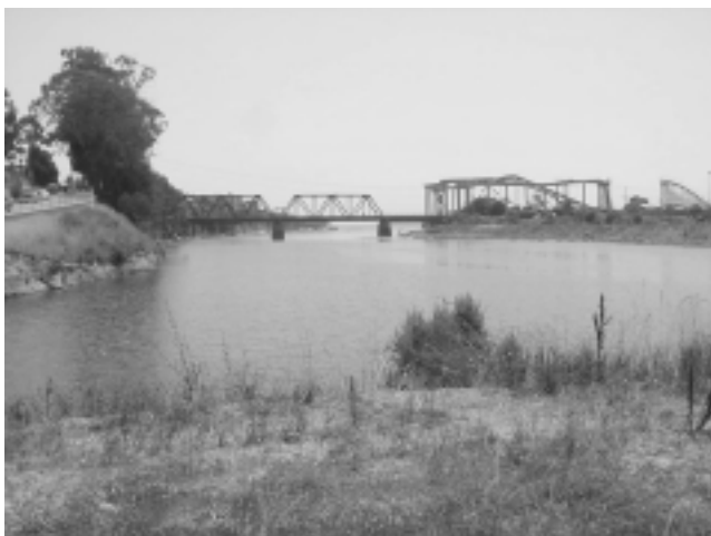
Figure 17 Trestle Bridge Focus Site
