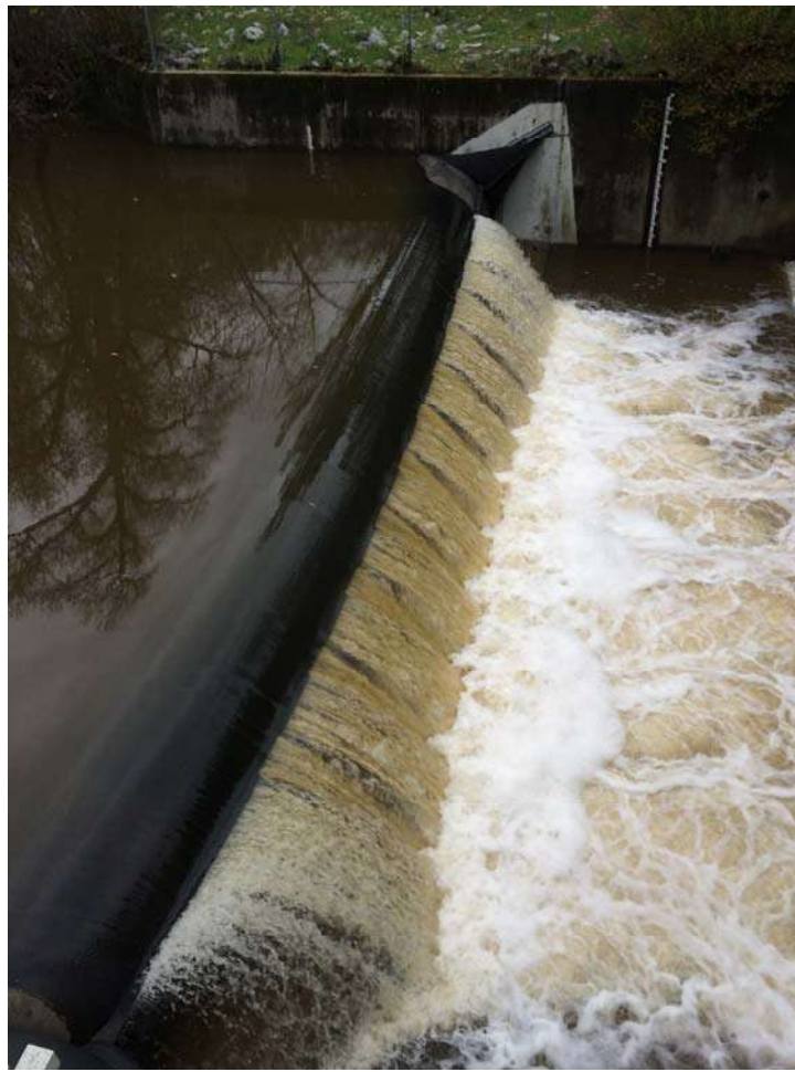
Felton Diversion, Inflatable Dam
