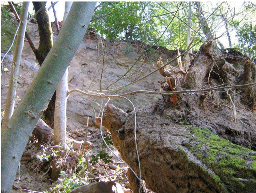
Landslide along Newell Creek Pipeline
