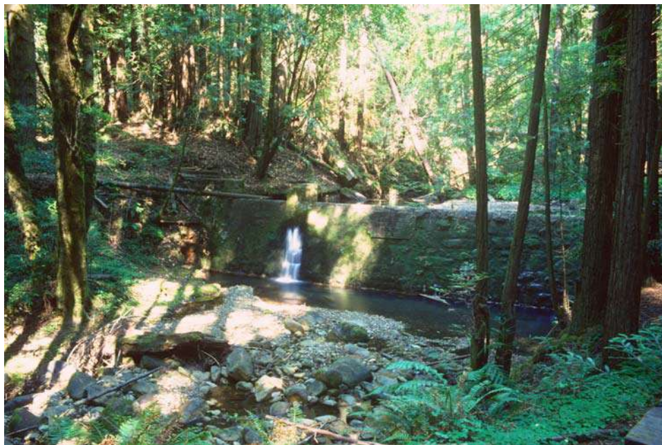
Creek Diversion Structure
