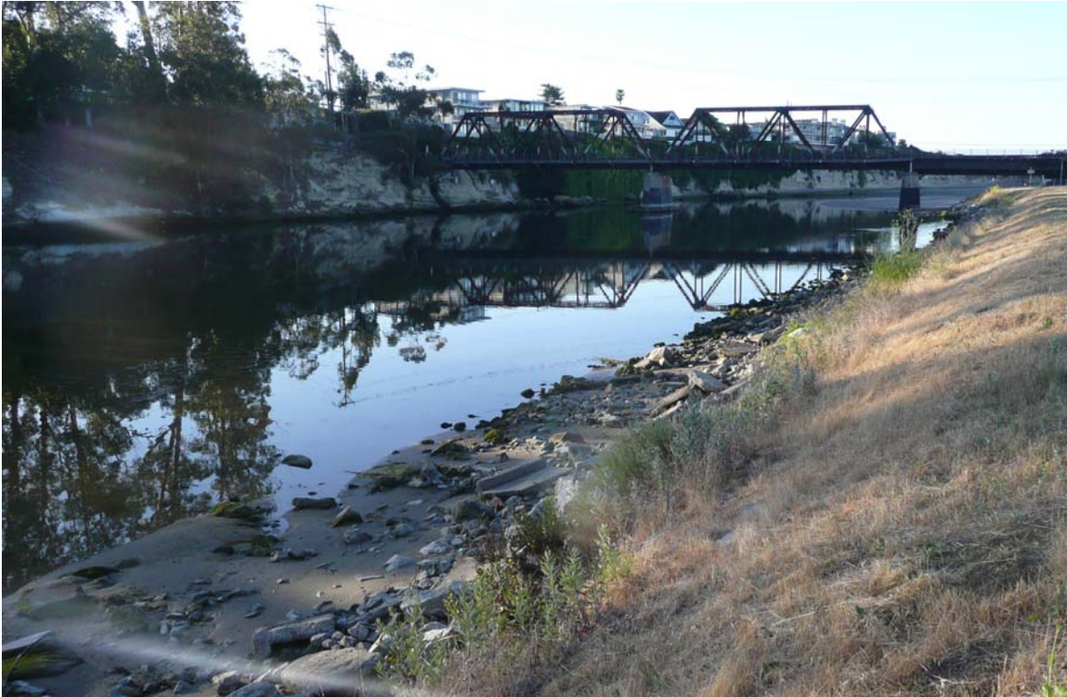
Figure 10. San Lorenzo River lagoon between trestle and water quality buoy, June 7, 2012.
