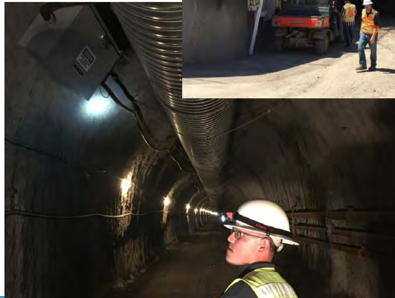
Photos from recent tunnel tour, Oakdale CA
