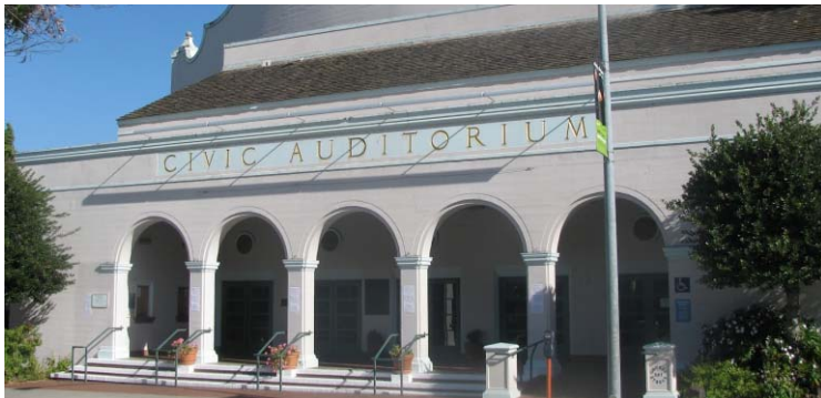
Civic Auditorium Roof Repair
