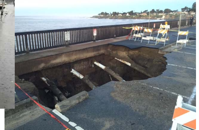
Seabright Beach Metal Pipe Replacement
