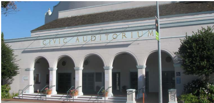
Civic Auditorium Roof Repair
