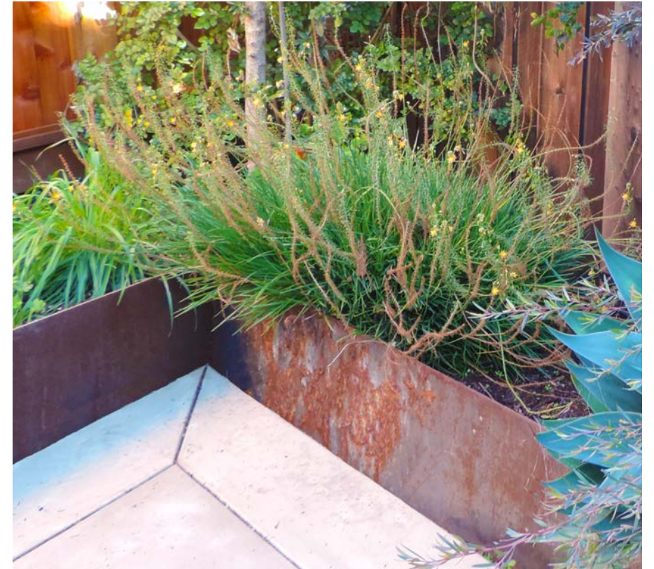
RAISED CORTEN STEEL PLANTER (photo by JLJA)
