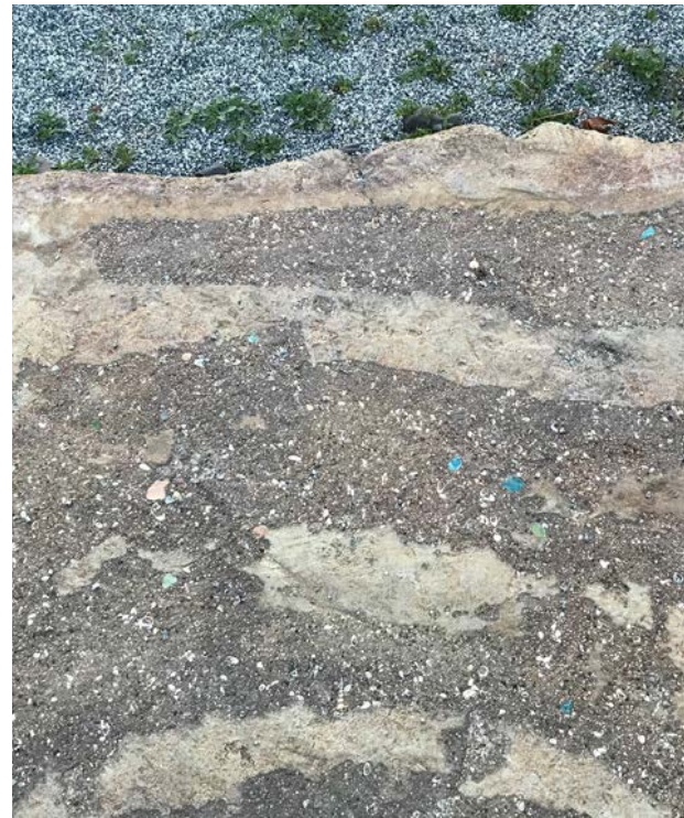
CONCRETE PAVING TO RESEMBLE SAND - West Cliff Bicycle Path, Santa Cruz (photo by JLJA)
