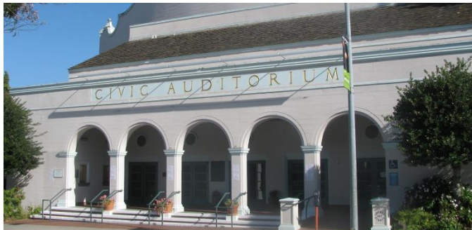
Civic Auditorium Roof Repair
