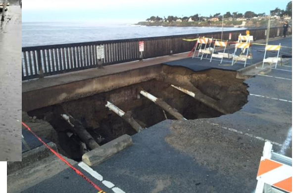
Seabright Beach Metal Pipe Replacement
