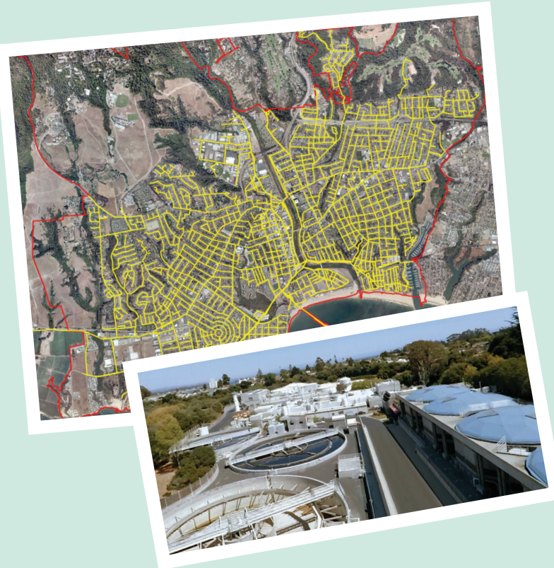
The City of Santa Cruz wastewater collections system consists of 160 miles of pipe supported by 21 pump stations leading to the Wastewater Treatment Facility.
