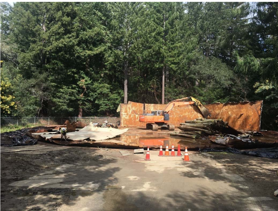
Figure 4 – Demolition of University Tank No. 5 in Preparation for Replacement
