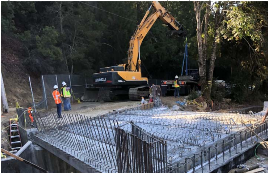
Figure 2 – Construction for Newell Creek Dam Spillway Bridge Replacement Project
