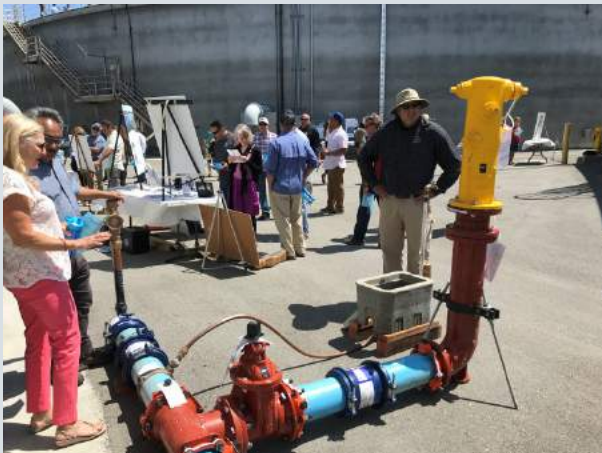
Water Distribution System Infrastructure
