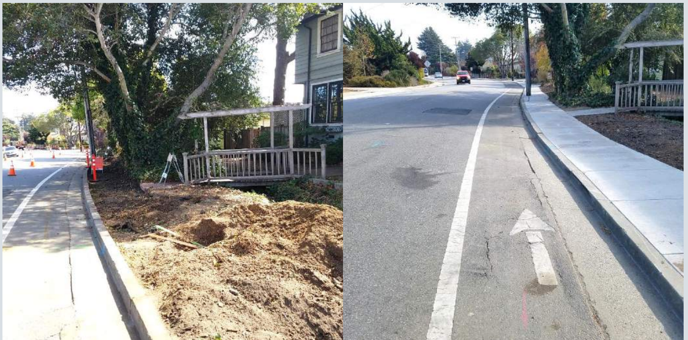
Bay Street Sidewalk Infill Project – Before and After
