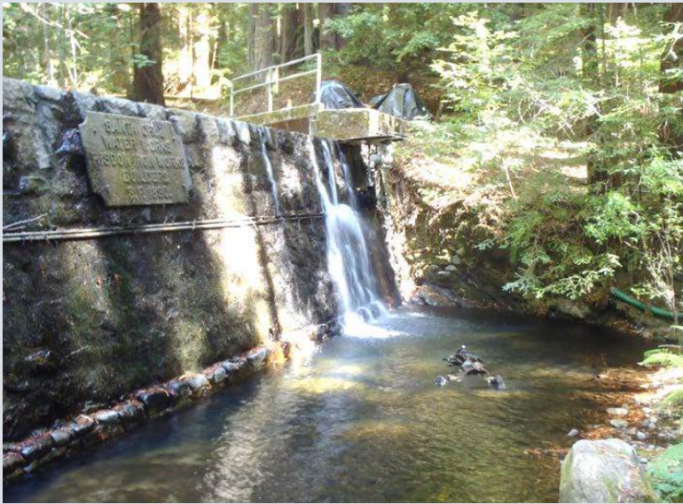
Laguna Diversion Dam
