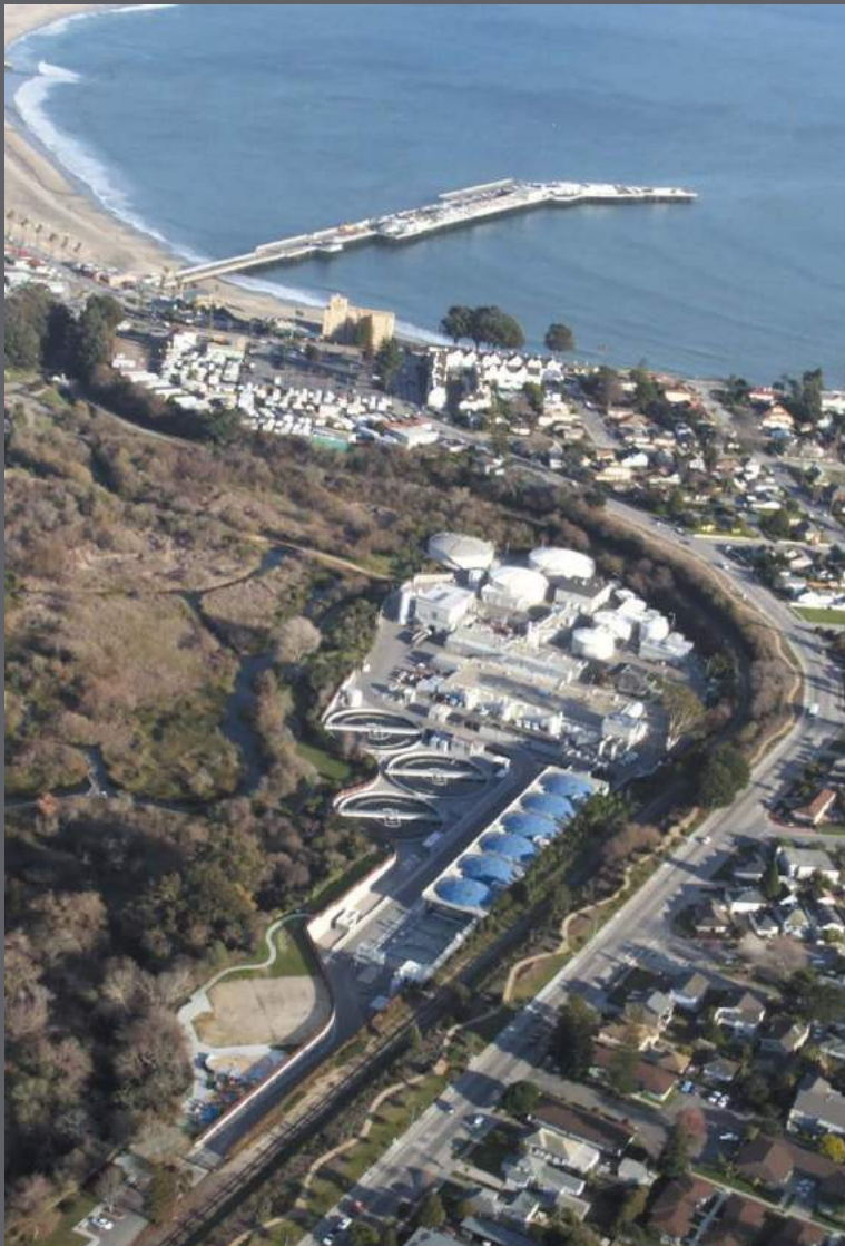
Aerial view of the Wastewater Treatment Facility
