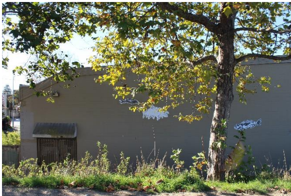
Figure 7: South half of east façade. Looking west.
