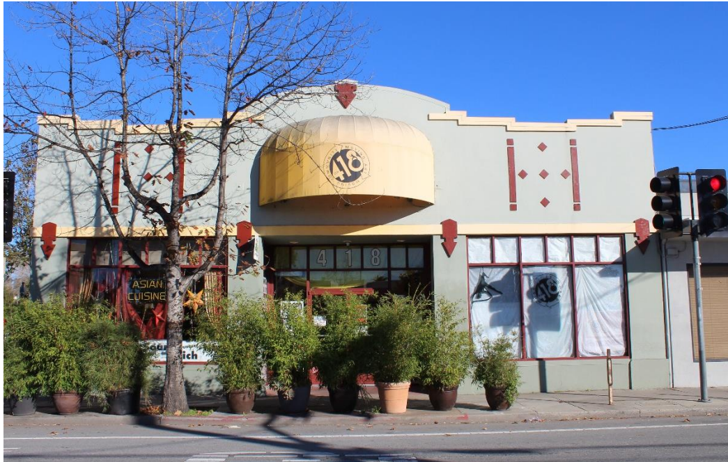
Figure 1: 418 Front Street, primary (west) facade. Facing east.
