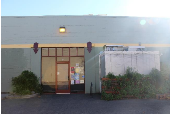
Figure 2: Metal framed entry with plate glazing inserted into north façade c. 1993. Looking south.
