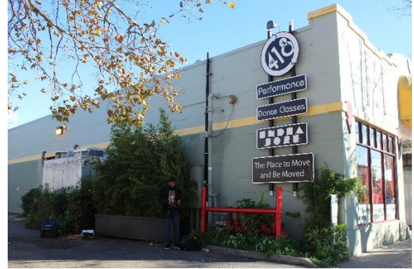
Figure 3: North façade. Looking southwest.
