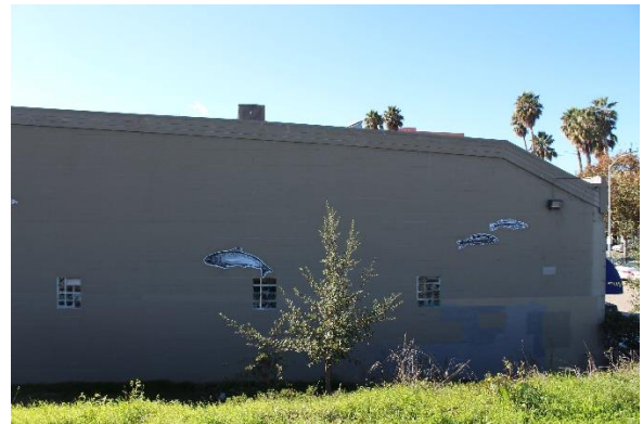
Figure 8: North half of east façade. Looking west.
