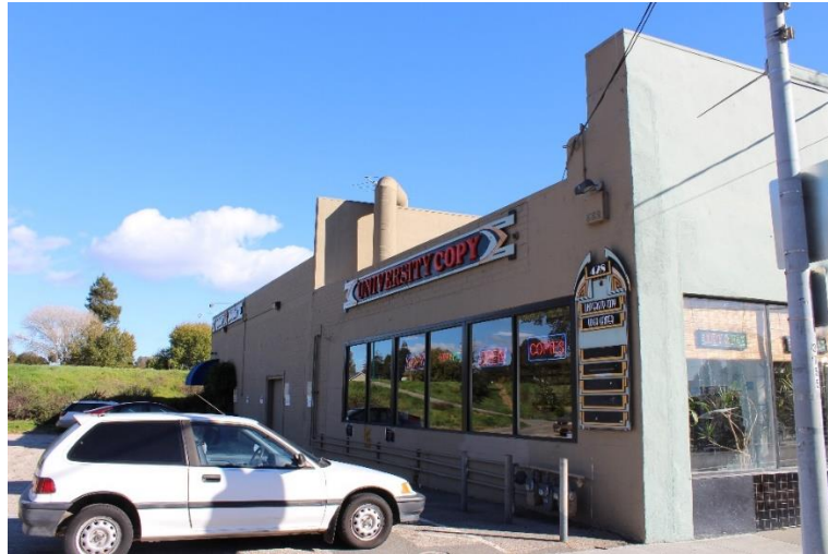
Figure 6: 428 Front Street, north façade. Facing southeast.
