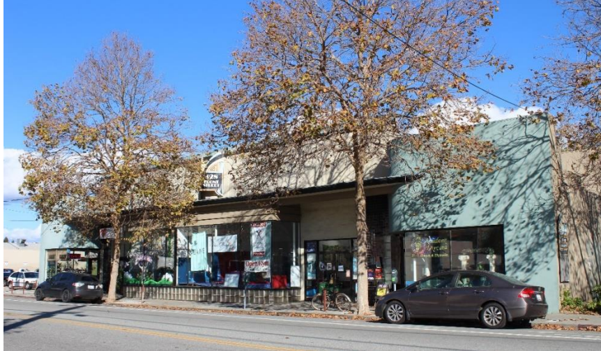
Figure 5: 428 Front Street, primary (west) façade. Facing east.
