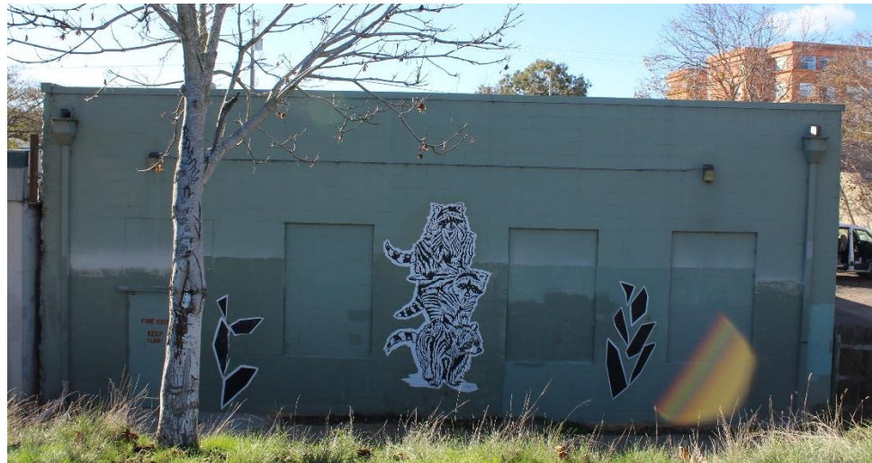
Figure 4: Rear (east) façade. Looking west.
