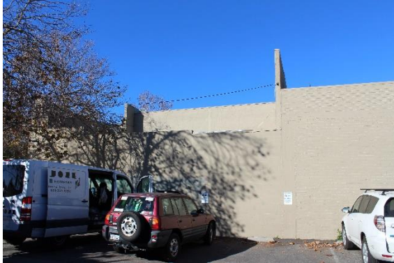
Figure 9: Western-half of south façade. Looking north.
