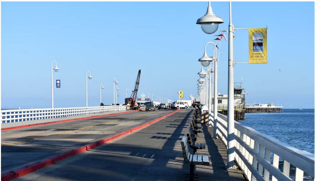
Existing View from Wharf Entrance
