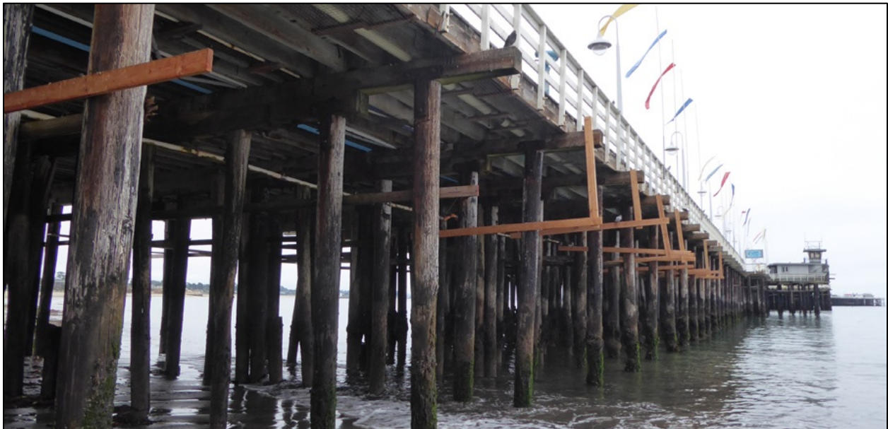
FIGURE 3. Santa Cruz Municipal Wharf Structure
