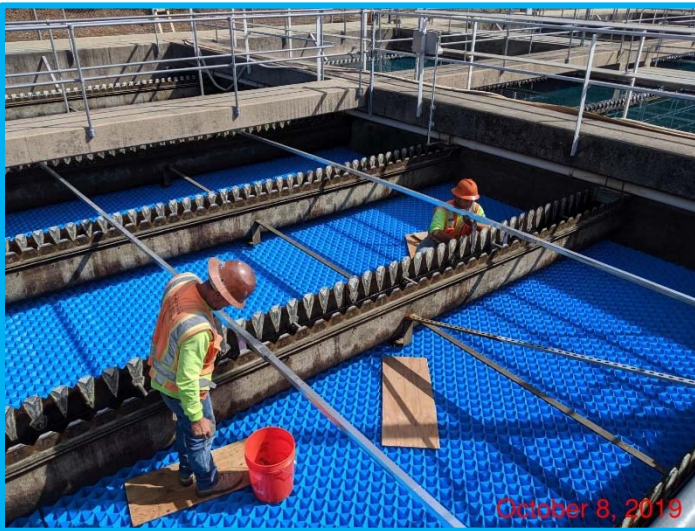
Figure 9 – GHWTP Tube Settler Installation
