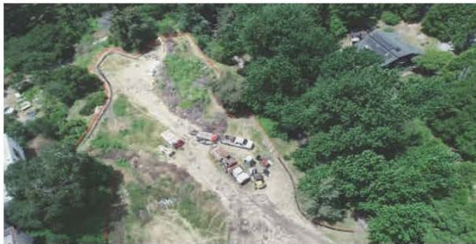
Riverbank Filtration drilling site.
