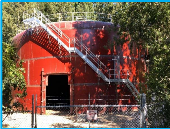
Figure 1 – University Tank 5 Roof Construction
