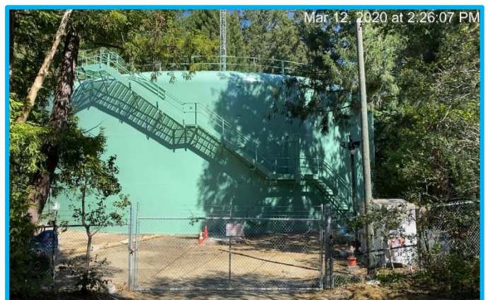
Figure 4 – University Tank 5 Final Paint
