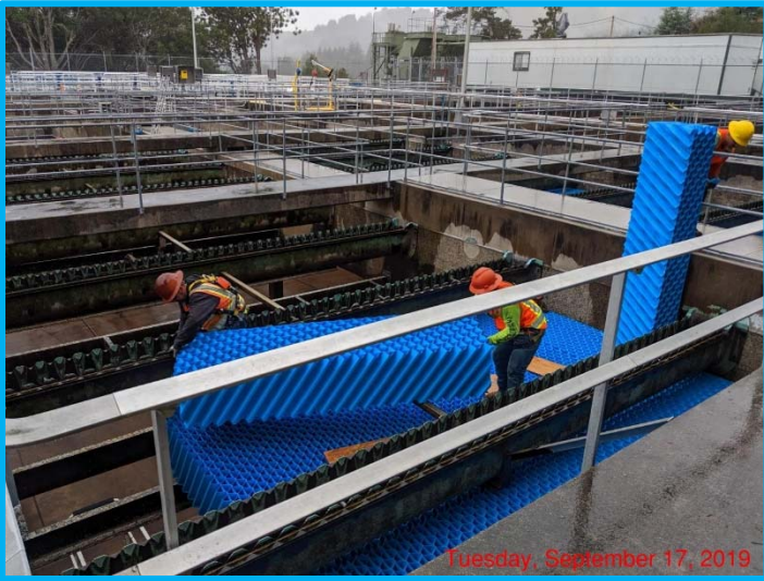
Figure 7 – GHWTP Tube Settler Installation
