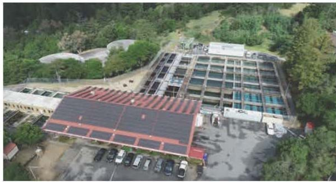
Graham Hill Water Treatment Plant
