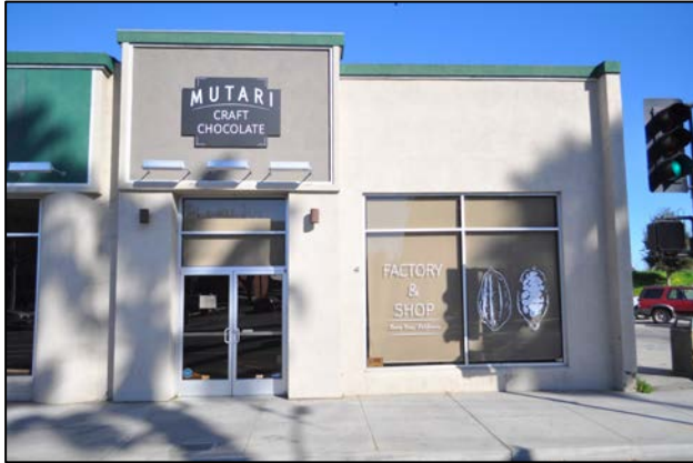
Figures 6 and 7. Left image details the new storefront installed in 2004. Comparison with Figure 8 below reveals that the entrances, fenestration and stucco parapet detailing are all new to the building. Right image details the rear elevation of the circa-1957 building (arrow).
