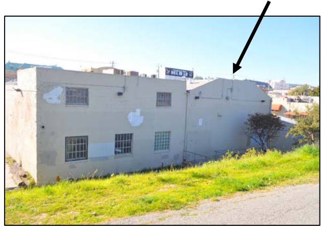
Figures 2 and 3. Left image shows the front (west) and primary elevation, with two-storefront configuration that completely modified the building's primary elevation in 2004. Right image details the rear elevation, showing the construction detailing of the first structure (circa-1939: arrow) and second structure (circa-1957), with multiple-pane aluminum frame windows.
