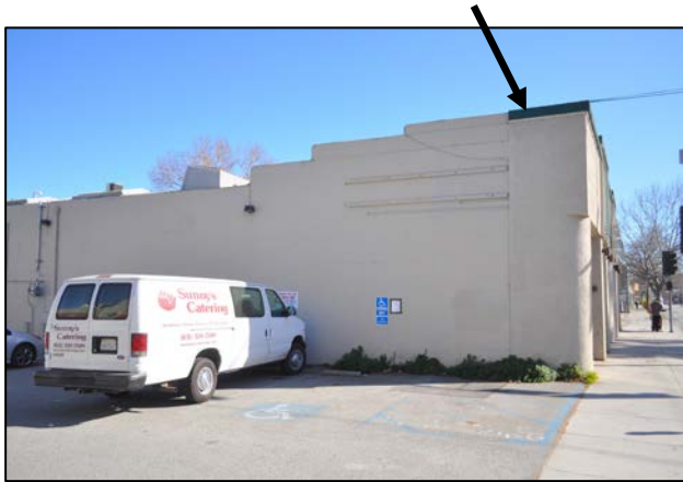
Figures 4 and 5. Left image shows the north elevation of the circa-1939 structure. The 2004 stucco detailing and new stucco wall cladding wraps around the building corner, modifying the original look of the building (arrow). Right image details the circa-1939 building's rear elevation, which does not contain any windows.
