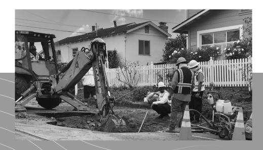
**Left:** Crews work to fix water main leak on Prospect Street
