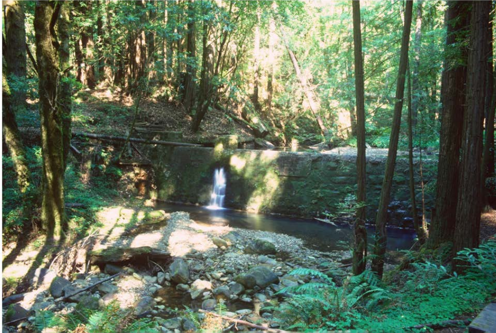
Figure 6-4. Laguna Creek Diversion Dam
