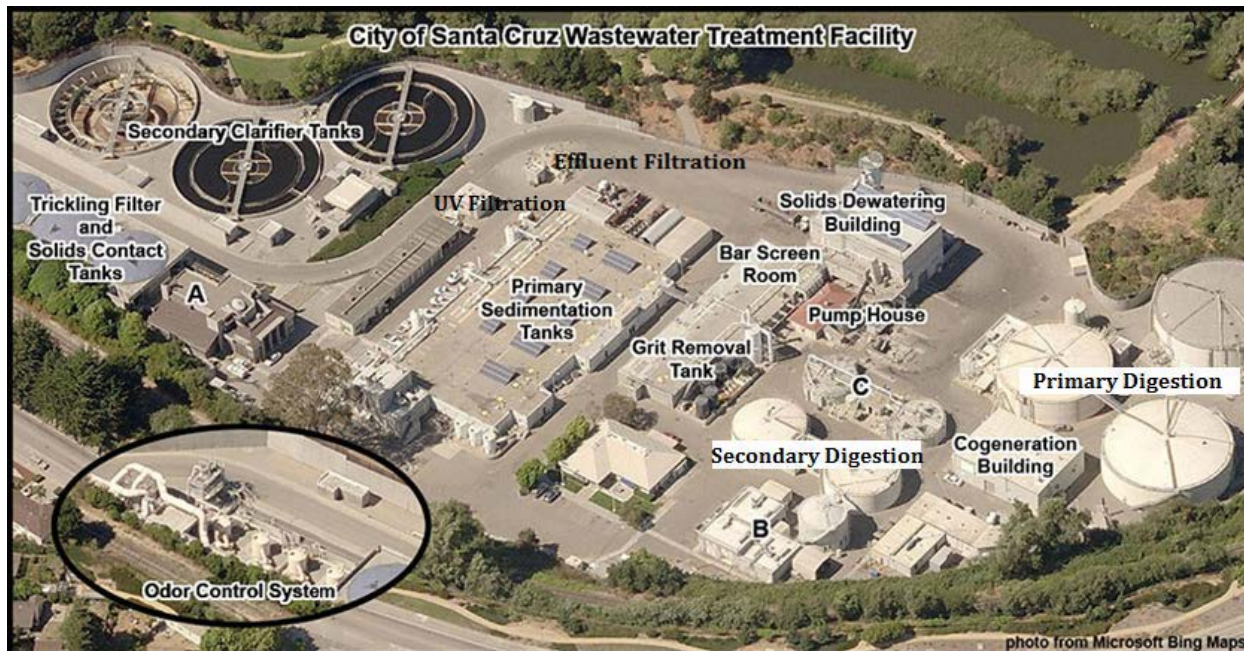
Figure 6-9. City of Santa Cruz Wastewater Treatment Facility
