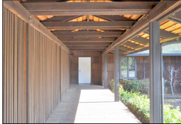
Figure 2. Looking east through veranda toward entrance.
