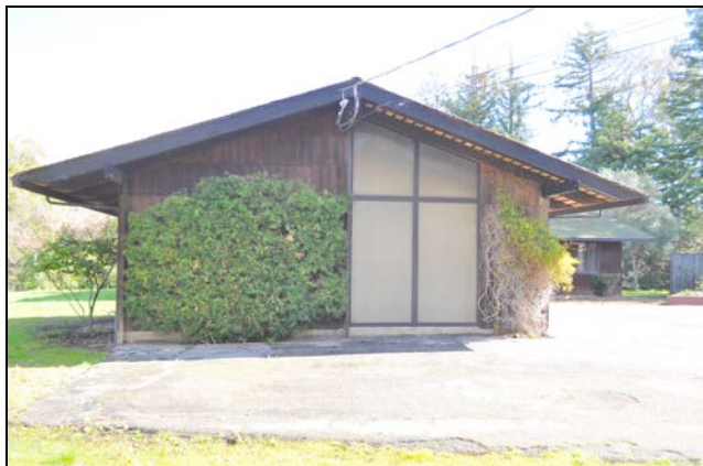
Figure 6. West elevation at garage, showing glazing resembling a Japanese Shoji screen.
