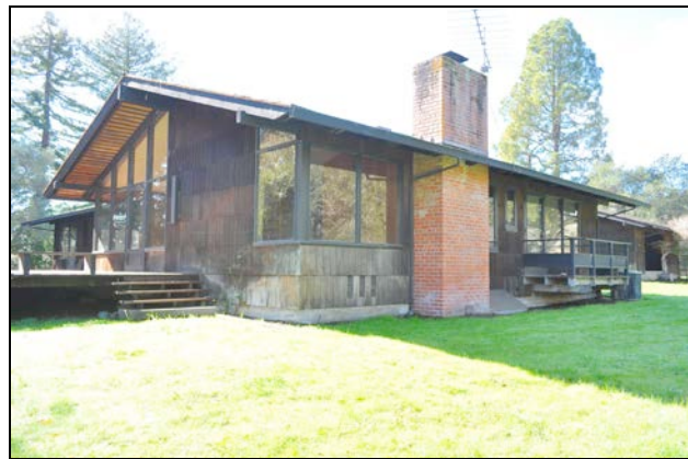
Figure 4. Rear (north) elevation at living room.
