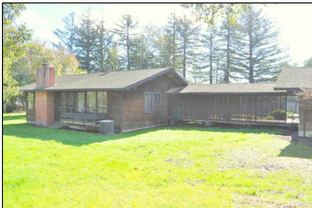
Figure 5. Rear (north) elevation, showing Japanese screen that connects the main house to the garage.
