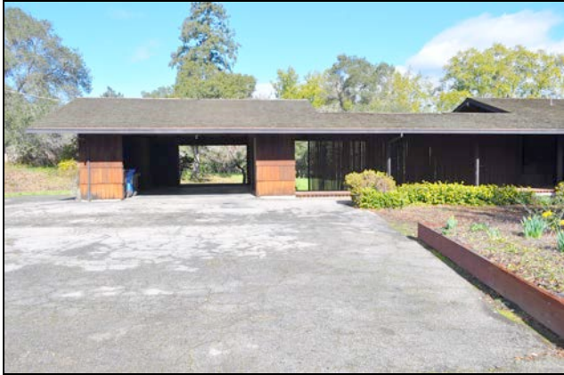
Figure 1. Garage and Japanese veranda, south elevation.
