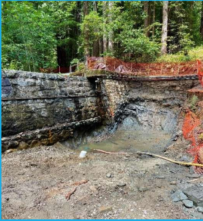
Photo 1: Laguna Dam Excavation
