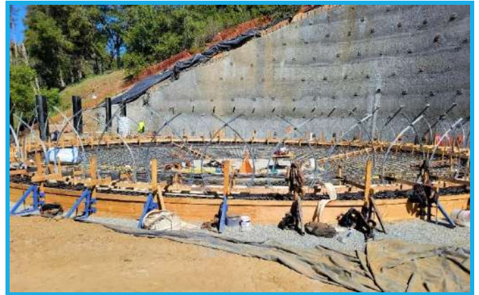
Photo 12: Residual Tank: Looking at slab footing rebar and seismic wall anchors
