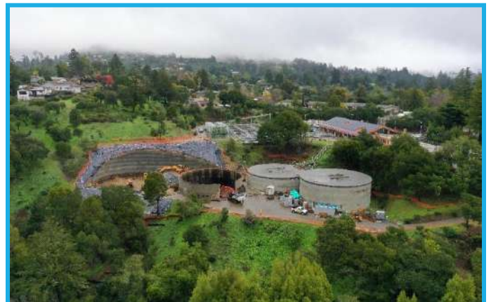
Photo 15: GHWTP Concrete Tanks Replacement Project – Solids Tank Demolition
