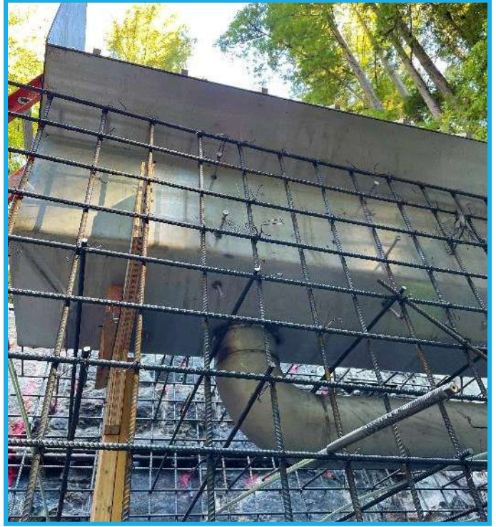
Photo 2: Laguna Dam - Rebar cage installed for Coanda Intake Screen
