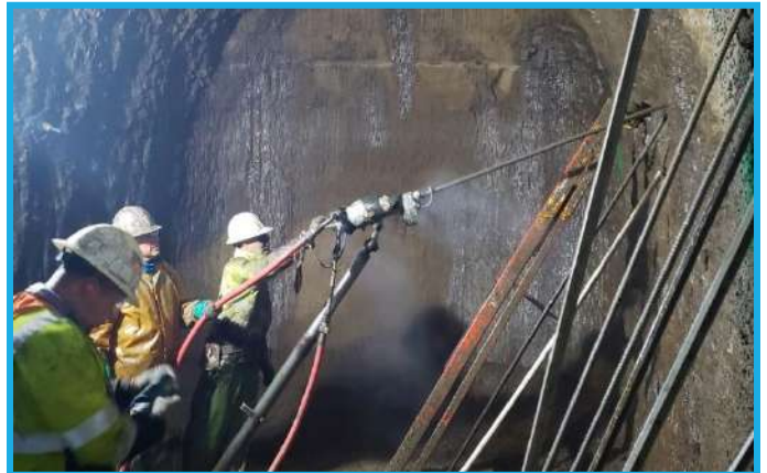
Photo 7: Newell Creek Dam Inlet/Outlet Project – Probe drilling prior to mandatory grouting
