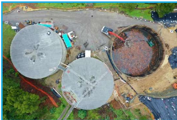
Photo 14: GHWTP Concrete Tanks Replacement Project – Solids Tank Demolition
