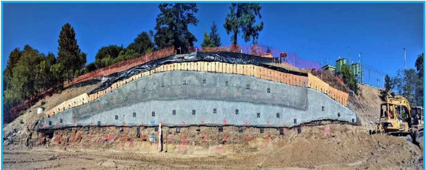
Photo 13: GHWTP Concrete Tanks Replacement – Soil nail wall at 3 rd lift
