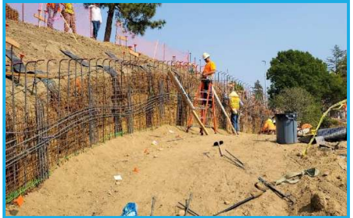
Photo 9: GHWTP Concrete Tanks soil nail wall rebar work
