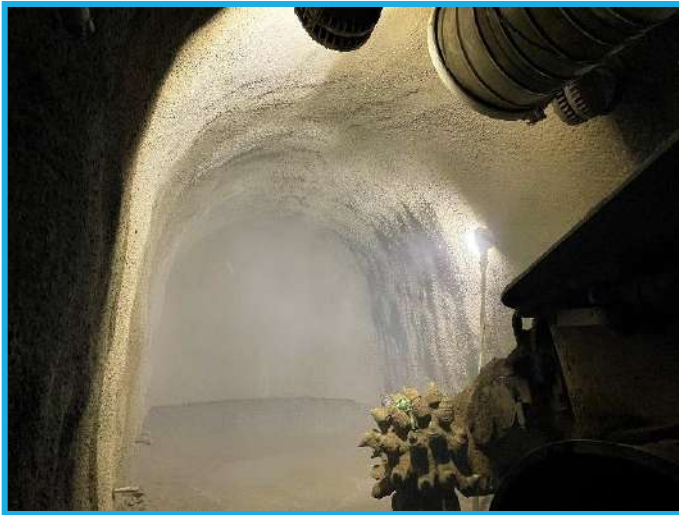
Photo 8: Newell Creek Dam I/O Replacement Project – Roadheader in tunnel near Sta 22+67
