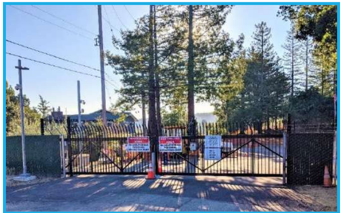
Photo 19: New entry gates in the closed position from the outside
