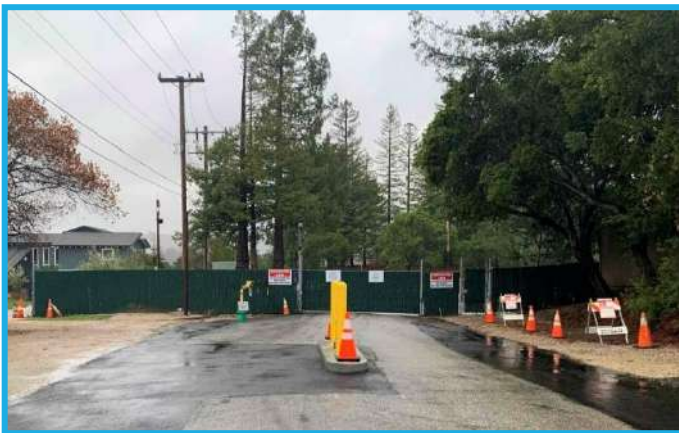
Photo 18: Entrance driveway with new island and final paving
