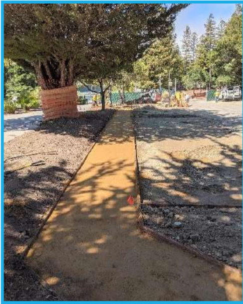
Photo 16: New pedestrian path on outside of GHWTP entry gate
