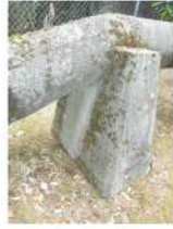
Figure 2-4. Exposed Pipe Support
