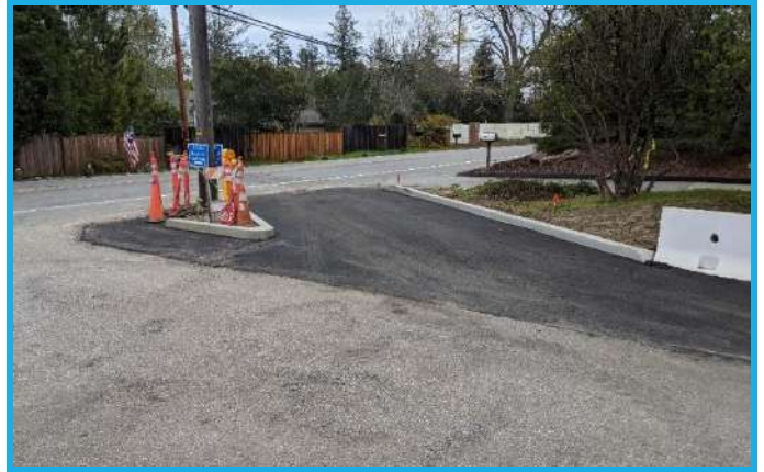
Photo 17: New right turn exit lane from GHWTP with final pavement
