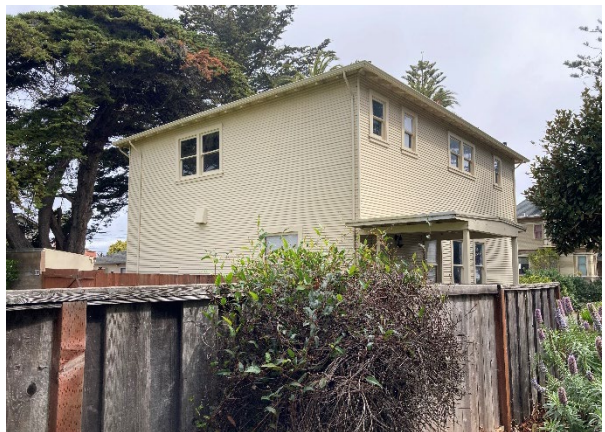
Figure 4: View of the rear of the carriage house, looking northeast.
