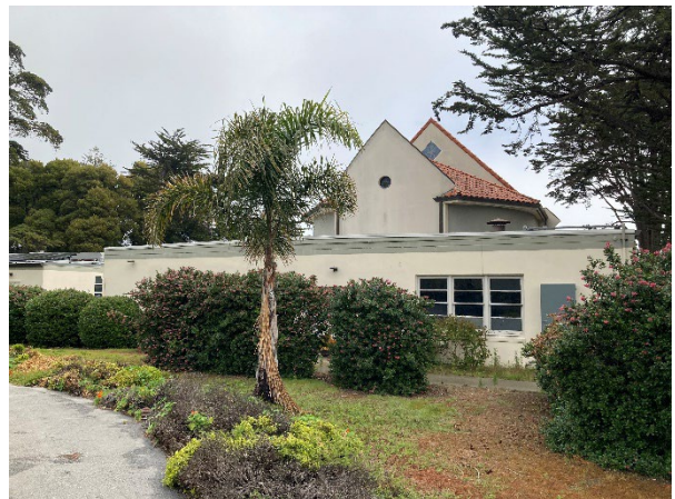
Figure 9: Rear façade of the Shrine, looking east.
