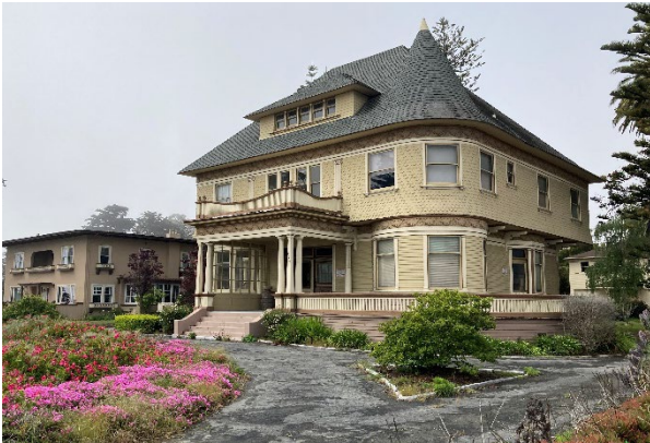
Figure 1: Rutherglen Terrace, with the Davis House in the left background, looking southwest.
