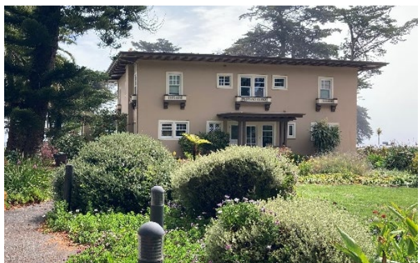
Figure 6: Rear façade of the Davis House, looking east.
