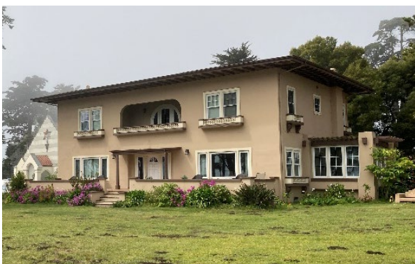
Figure 5: Davis House, primary façade, looking southwest.
