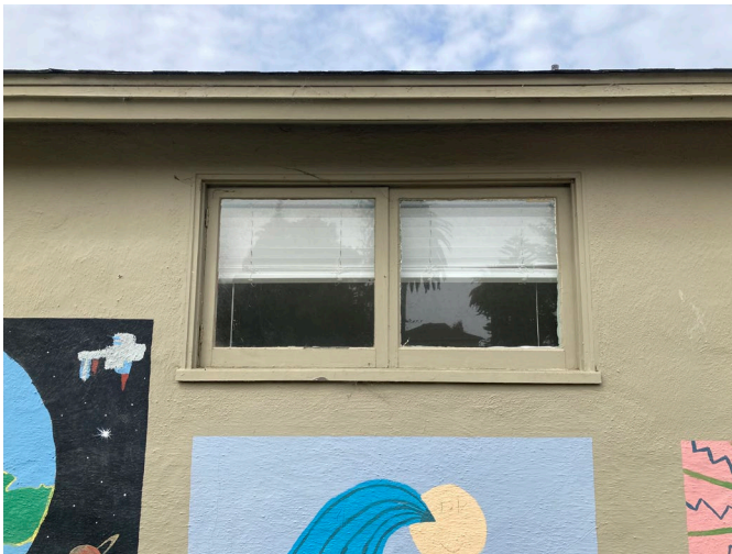
Figure 3: Typical wood casement window at the east façade, looking west.
