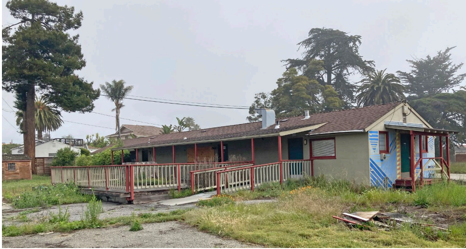
Figure 2: Oblique view of the west (left) and south (right) façades, facing northeast.
