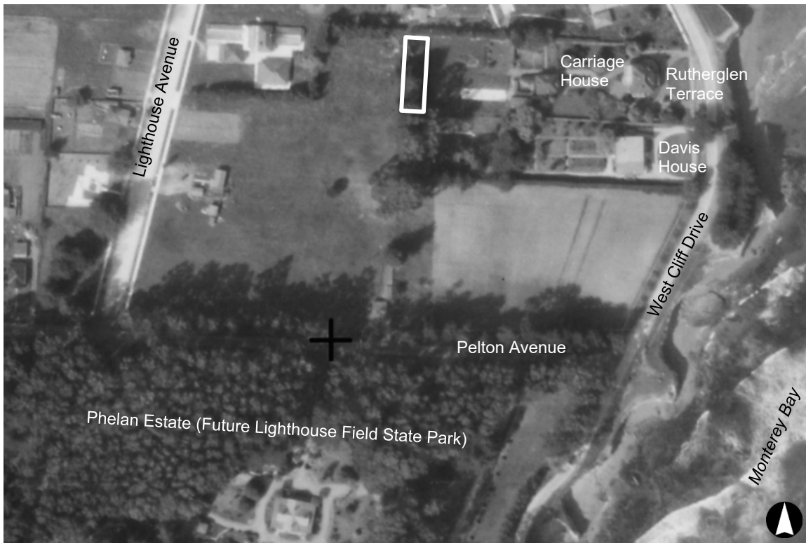
Figure 14: Aerial photograph showing the future location of the subject building (white rectangle) and vicinity, March 13, 1931. Fairchild Aerial Surveys, Flight C-1437, Frame B-37. UC Santa Barbara Special Collections. Edited by Page & Turnbull.
