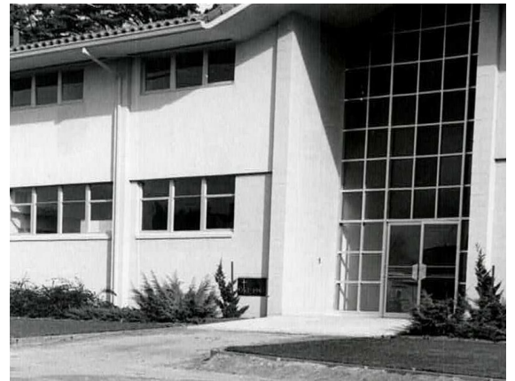
Figure 30: Detail view of the main entrance area, January 1964. Source: Courtesy Oblates of St. Joseph.
