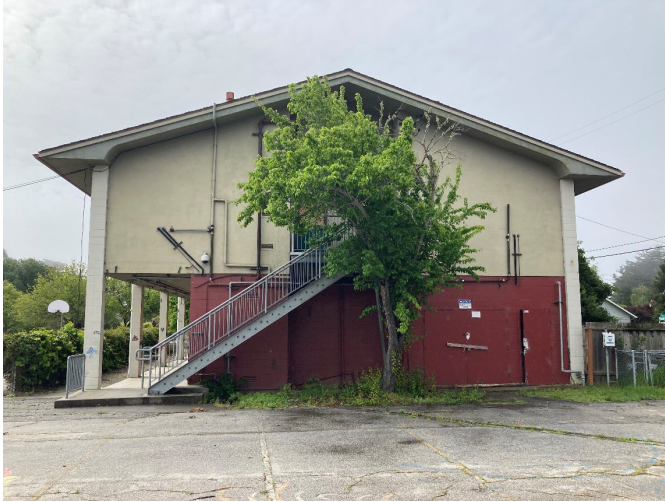
Figure 5: North façade, facing south.
