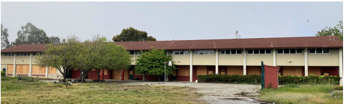
Figure 7: East façade, looking west.
