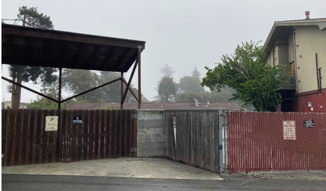
Figure 13: View of the north gate and adjacent garage enclosure structure.
