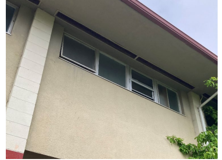
Figure 10: Typical fenestration at second story of east façade, looking northwest.
