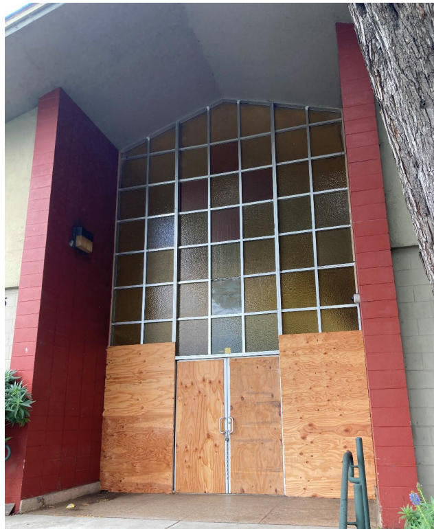
Figure 4: Double-height main entrance at the primary façade.
