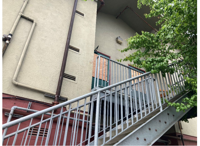
Figure 6: Detail of staircase and doors at the second story, looking southwest.
