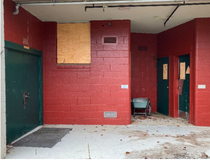
Figure 8: Recessed restroom entrances at the rear façade.
