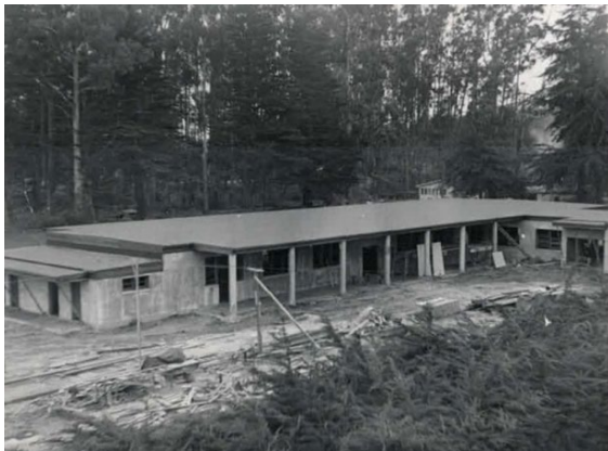
Figure 22: Original one-story chapel under construction in 1951. Source: Oblates of St. Joseph, online.
