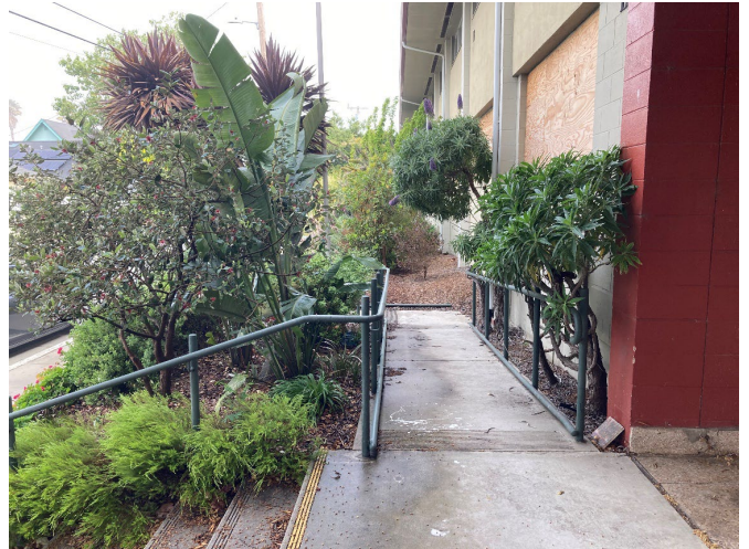
Figure 3: Ramp to main entrance, looking north.
