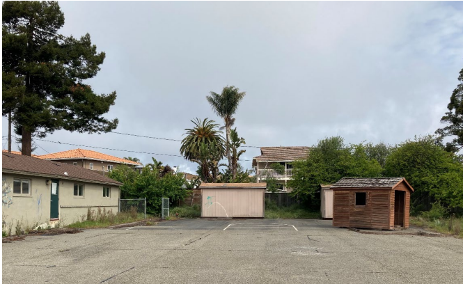
Figure 15: Prefabricated sheds located near the north perimeter of the site, immediately east of the former refectory building, looking north.
