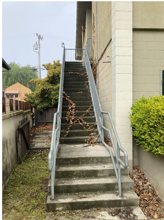
Figure 11: Concrete stairs with metal railings at the south façade, looking west.
